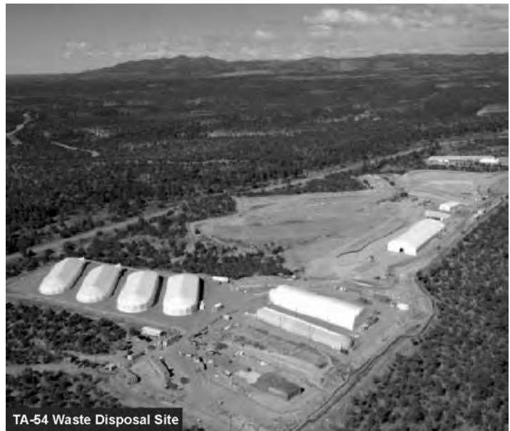
TA-54 Waste Disposal Site
