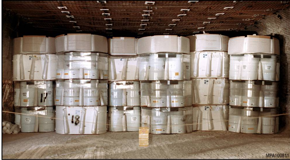
FIGURE 4.1.4-2 Disposal of Contact-Handled Transuranic Waste in Typical 208-L (55-gal) Drum 7-Packs at WIPP (bagged magnesium oxide chemical buffer is on top of each stack) (Source: DOE 2007)
