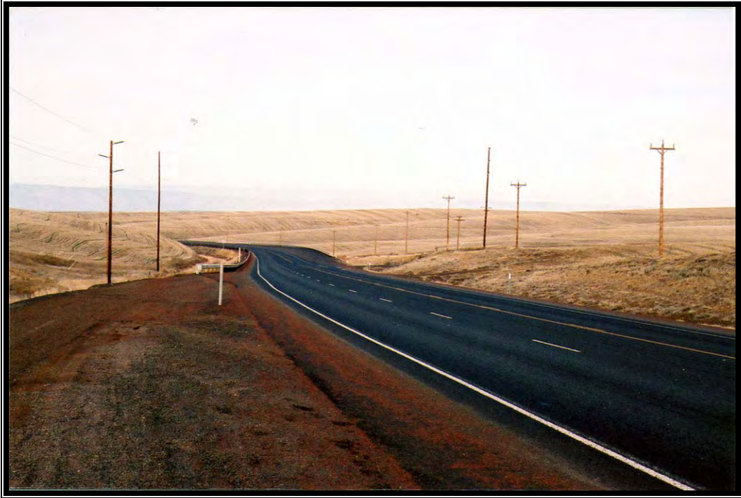
PHOTO 9: US 97 at MP 12 looking north.
