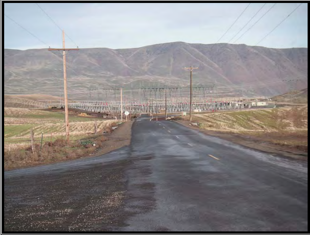
PHOTO 1: John Day Substation looking north.
