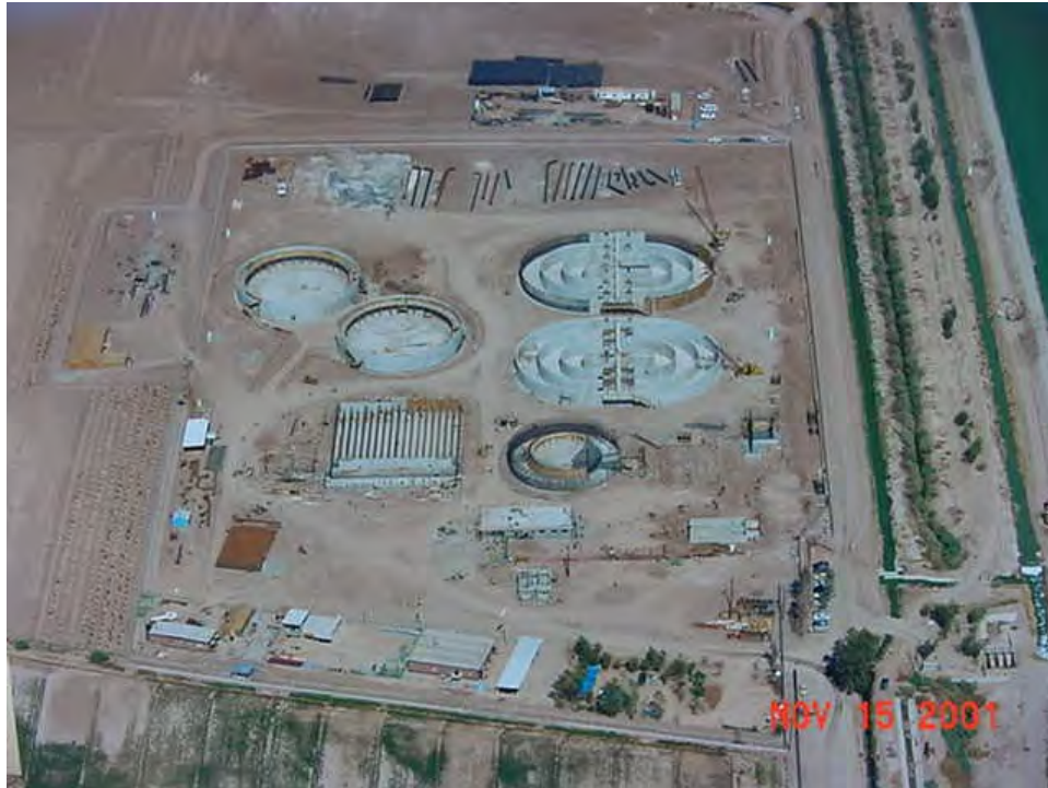
FIGURE L-10 Aerial View of the LRPC Sewage Treatment Plant next to the Zaragosa Oxidation Lagoons during Construction (November 2001)
