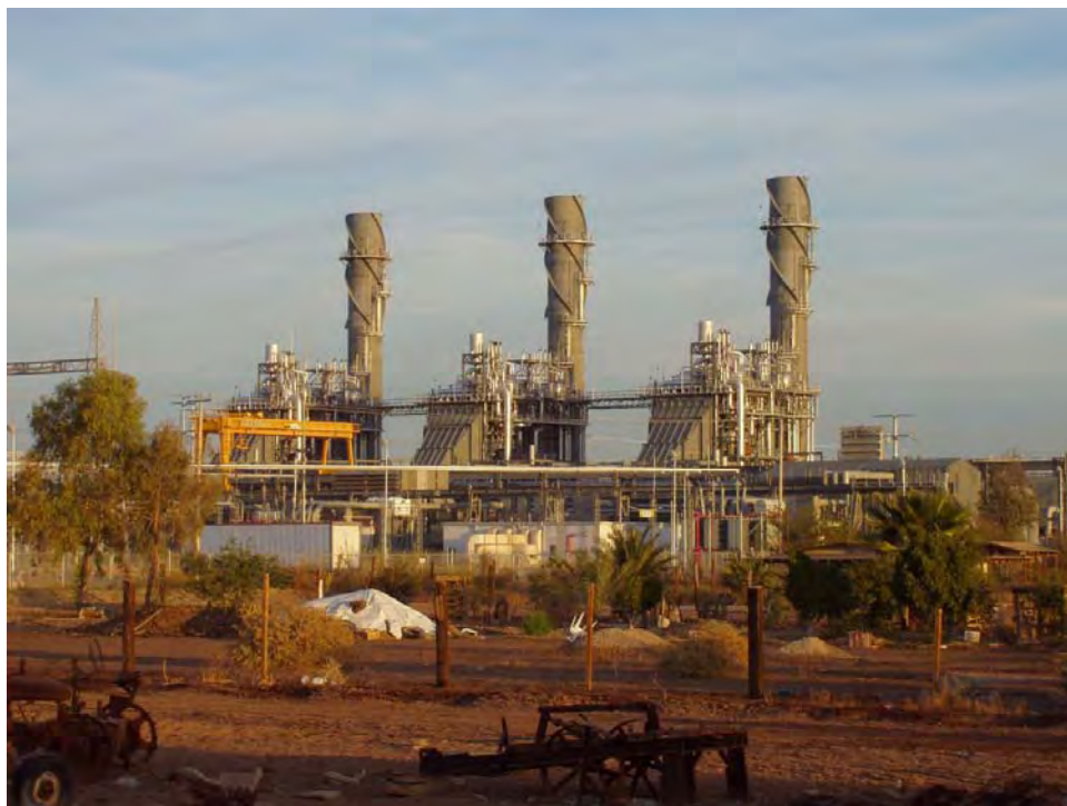
FIGURE L-7 View of the EAX Unit from the Field
