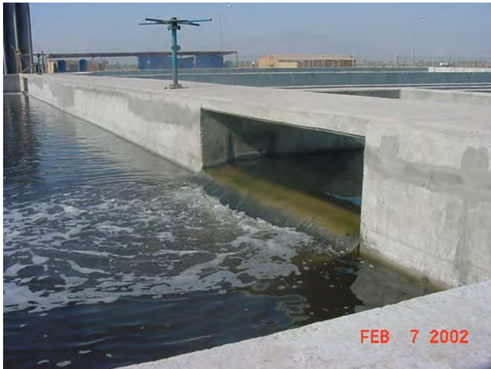
FIGURE L-11 Overflow from the Disinfection Chamber to the Gray Water Pump Well
