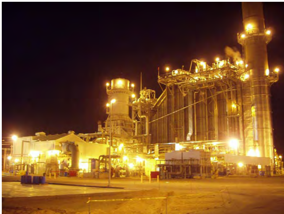
FIGURE L-9 View of the EBC Unit at Night
