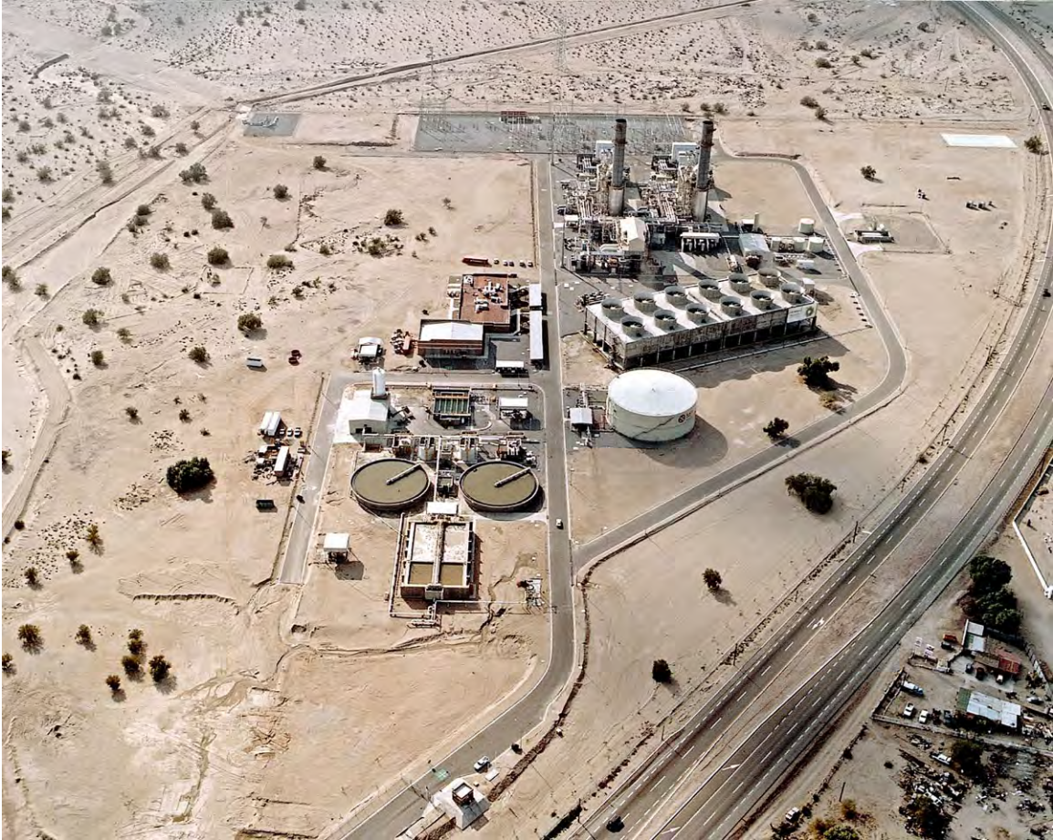
FIGURE L-1 Aerial View of the TDM Power Plant (North is to the right of the photograph. The facility property totals approximately 78.2 acres [31.7 ha]. The power plant and its facilities occupy approximately 26.8 acres [10.9 ha].)
