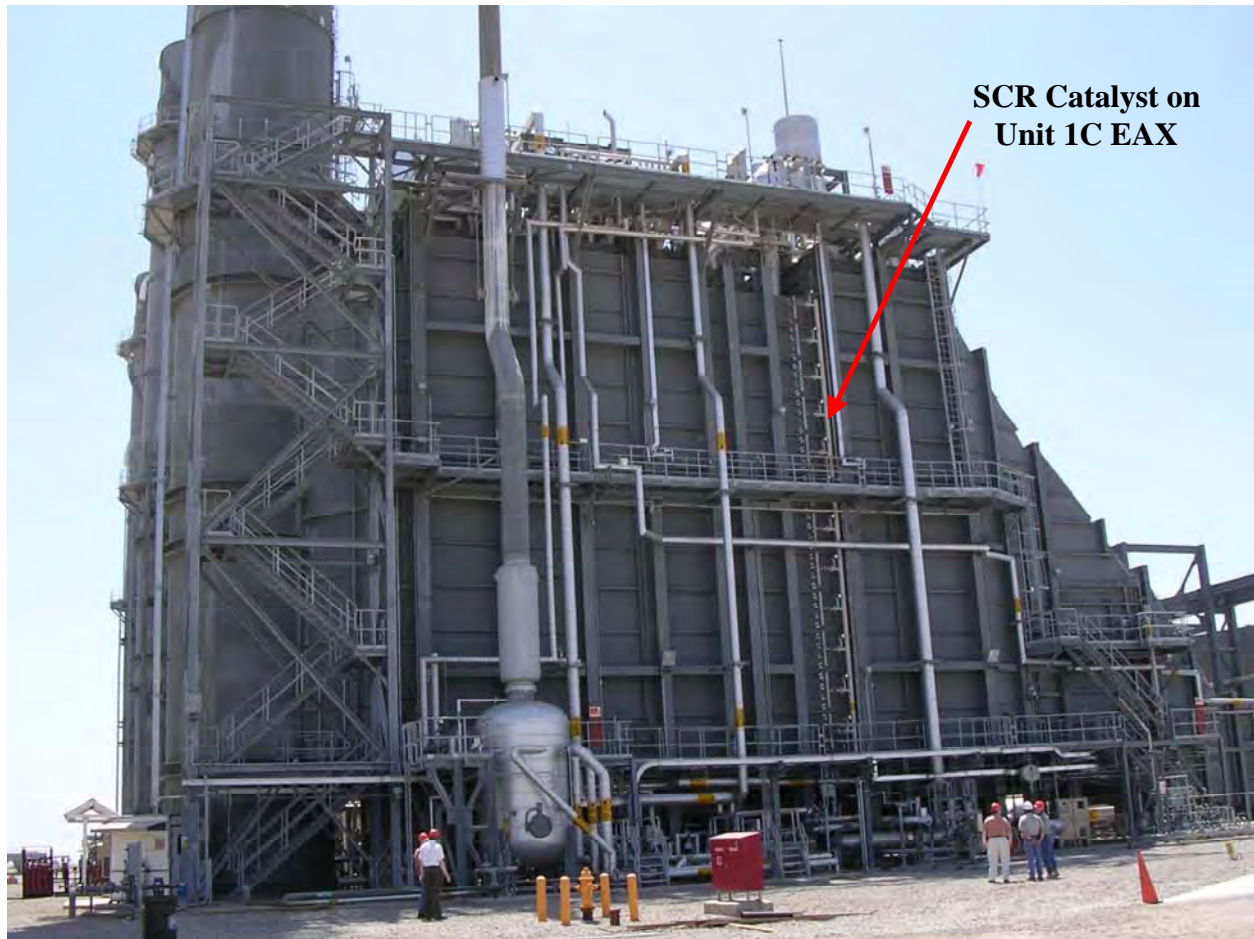
FIGURE L-5 View of EAX-1C Export Gas Turbine Showing the Location of the Selective Catalytic Reduction (SCR) System for NO x Control Installed in March 2004 (If an oxidizing catalyst was installed under Alternative 3, it would be retrofitted in the vicinity of the SCR catalyst.)
