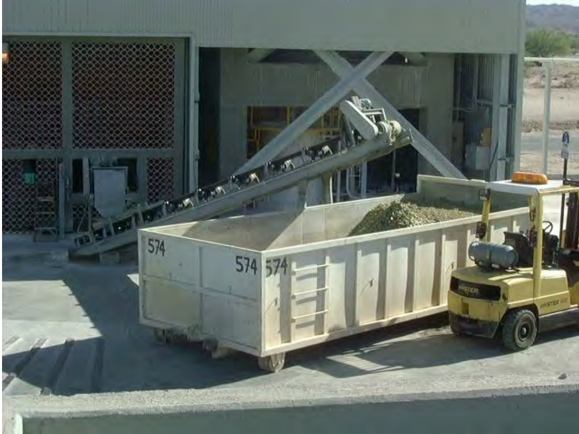
FIGURE L-4 View of Solids Removed from Sewage Treatment Processing at the TDM Facility (This is a view of the filter press house and the dump bin where solids are deposited for disposal in the solid waste landfill.)
