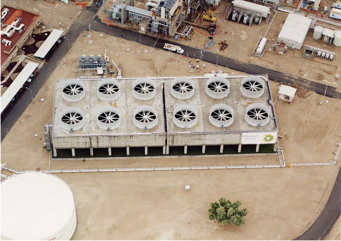
FIGURE L-2 Aerial View of the Cooling Tower (The cooling tower measures 350 ft [106.5 m] in length and 35 ft [41.1 m] in width, by 57 ft [17.4 m] in height. Each cooling fan measures 36 ft [11 m] in diameter. Note the truck on the road to the west of the cooling tower [north is to the right of the picture] for scale.)
