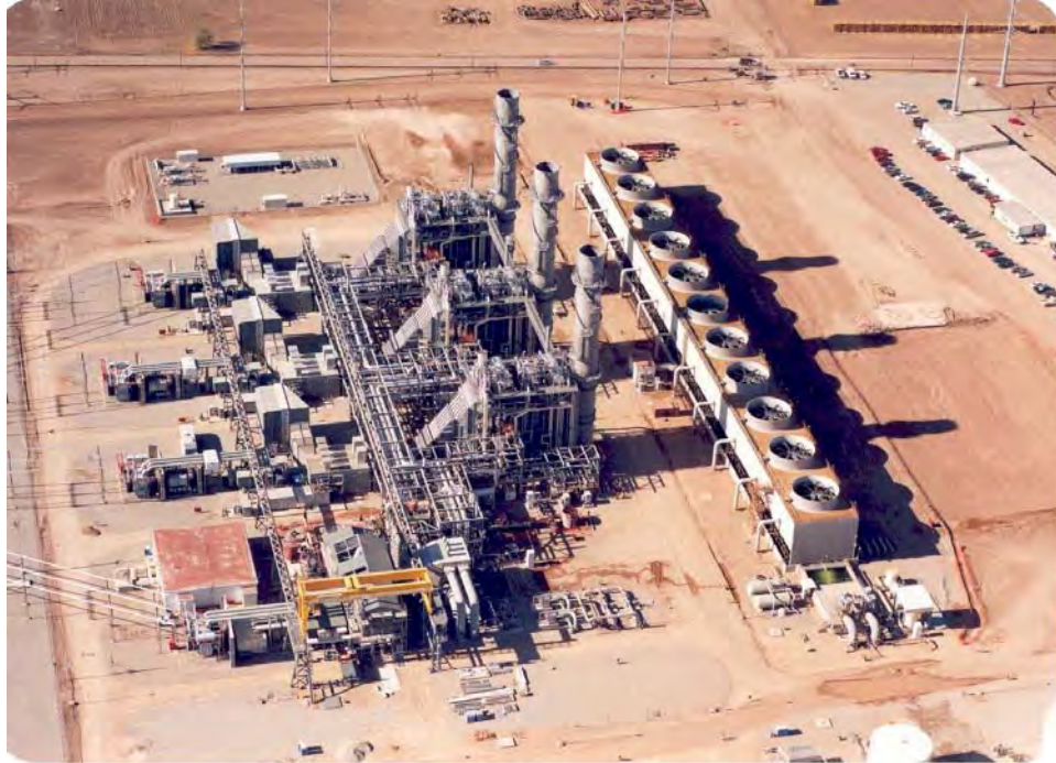
FIGURE L-6 Aerial View of LaRosita 1 (LR1), the EAX Unit (The 11-unit cooling tower is shown on the right and the three gas turbines on the left. Each of the gas turbines is equipped with a heat recovery steam generator that powers a single steam turbine in a combined-cycle mode.)
