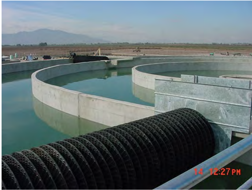
FIGURE L-12 Sewage Treatment Plant Aeration Tank
