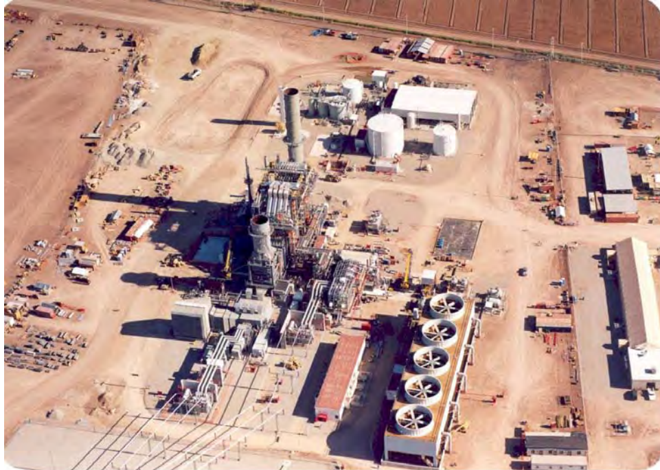
FIGURE L-8 Aerial View of LaRosita 2 (LR2), the EBC Export Unit (This unit consists of a single gas turbine and a single steam turbine operating in a combined cycle. The on-site water treatment plant is near the top of the picture.)
