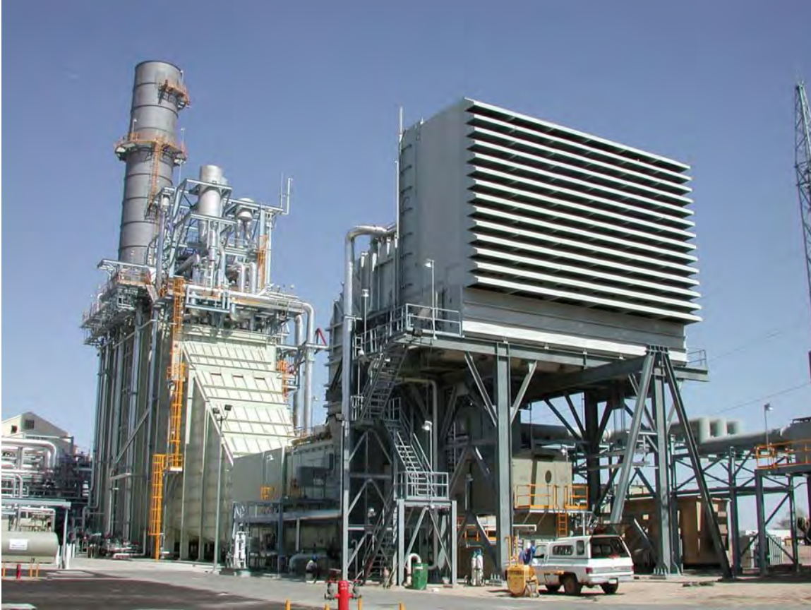
FIGUER L-3 View of Gas Turbine Inlet Air Structure, Gas Turbine, Heat Recovery Steam Generator, and Stack for One of the Two Units at TDM (The inlet air filter structure measures 69.5 ft [21.2 m] high from ground elevation, 44 ft [13.4 m] wide. The length of the turbine train front to back [from air filter structure to end of stack width] is 282 ft [86 m]. Note the pickup truck below inlet filters for scale.)
