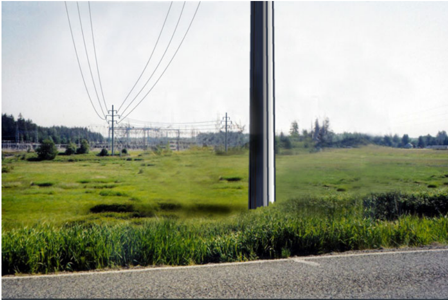
Looking east at Custer Substation from Blaine/Ferndale Road
