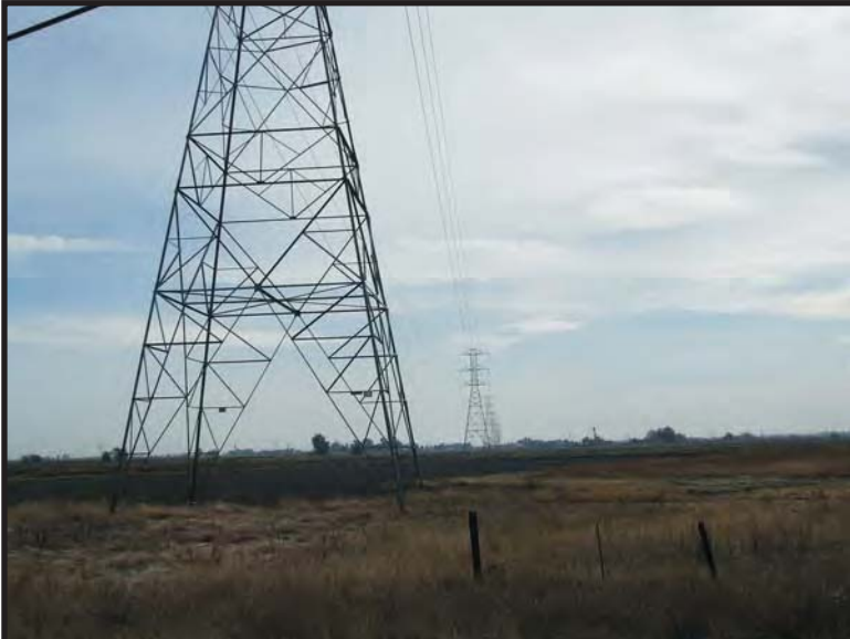
Photo 2C-1 (Alternative C): intersection of Keys Road and Pleasant Grove Road, facing southeast
