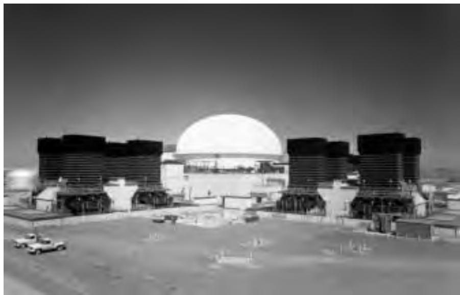
Figure 2–2 Fast Flux Test Facility
