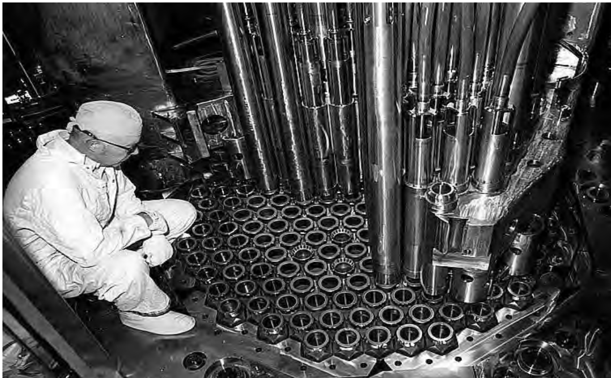
Figure D-6 Instrument Trees Over the Initial (Unfueled) Core
