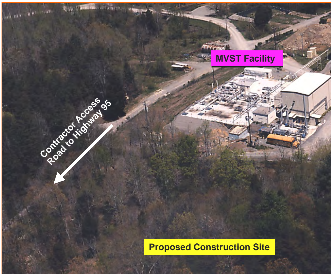
Figure 2-2. DOE would lease the Melton Valley Storage Tanks facility and an adjacent area of land to construct the waste treatment facility. The location is isolated from ORNL by Haw Ridge.
