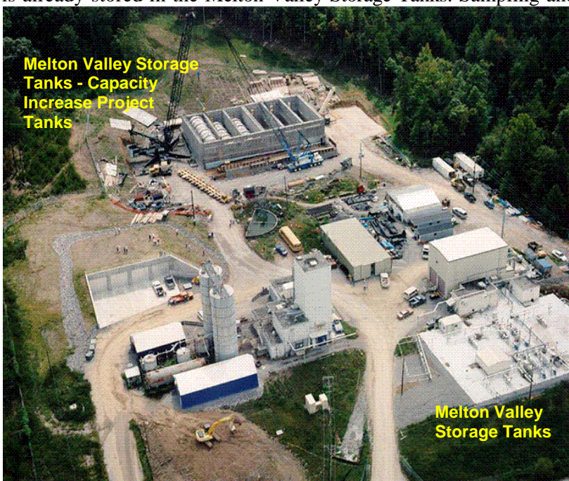
Figure S-2. Aerial view of the Melton Valley Storage Tanks—Capacity Increase Project during installation of the six 100,000-gallon tanks, which are located south of the eight 50,000-gallon Melton Valley Storage Tanks.
