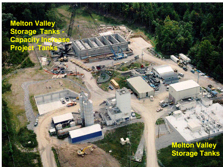
Figure 1-2. Aerial view of the Melton Valley Storage Tanks–Capacity Increase Project during installation of the six 100,000-gallon (gal) tanks located south of the Melton Valley Storage Tanks.
