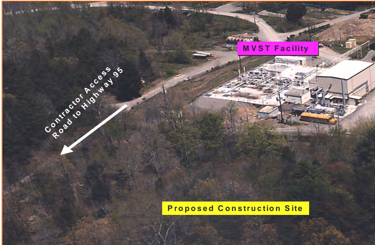
Figure S-4. DOE would lease the Melton Valley Storage Tanks facility and an adjacent area of land to construct the waste treatment facility. The location is isolated from ORNL by Haw Ridge.
