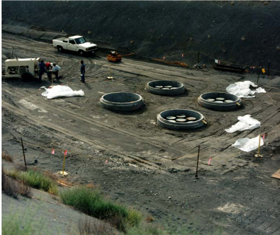
1 2 3 Figure 2.13. High-Intensity Containers in a Low-Level Waste Disposal Trench 4
