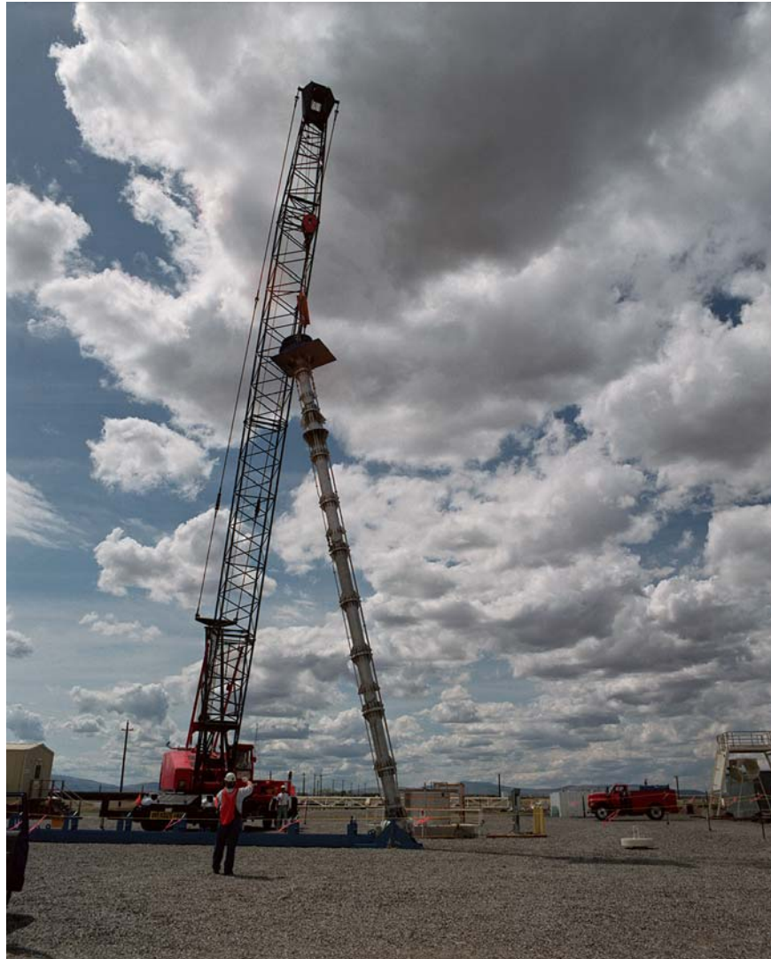
Figure 2.2. Long-Length Equipment Being Removed from a Tank
