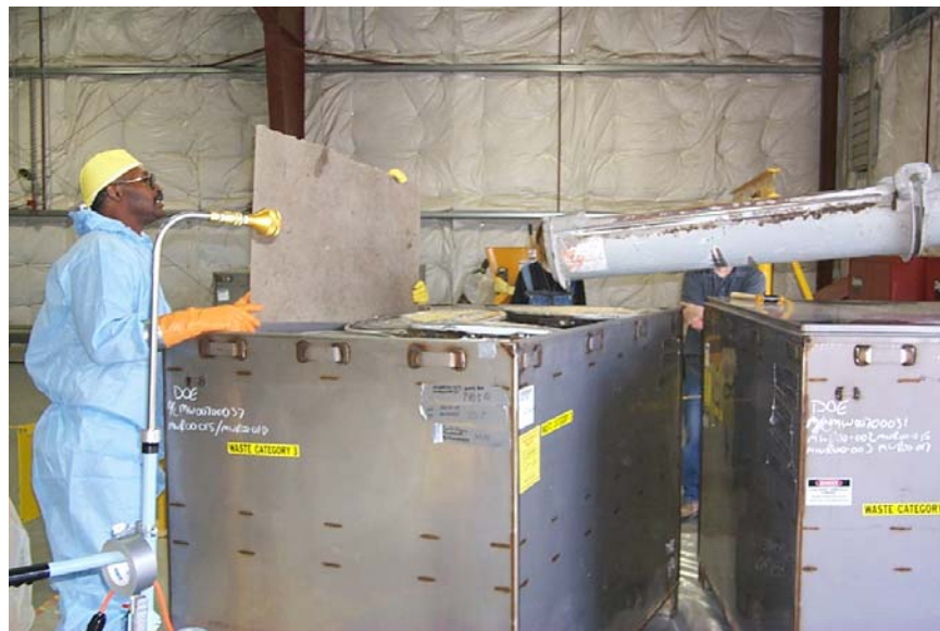
26 27 28 Figure 2.10. Macroencapsulation of Mixed Low-Level Waste Debris at a Local 29 Commercial Treatment Facility
