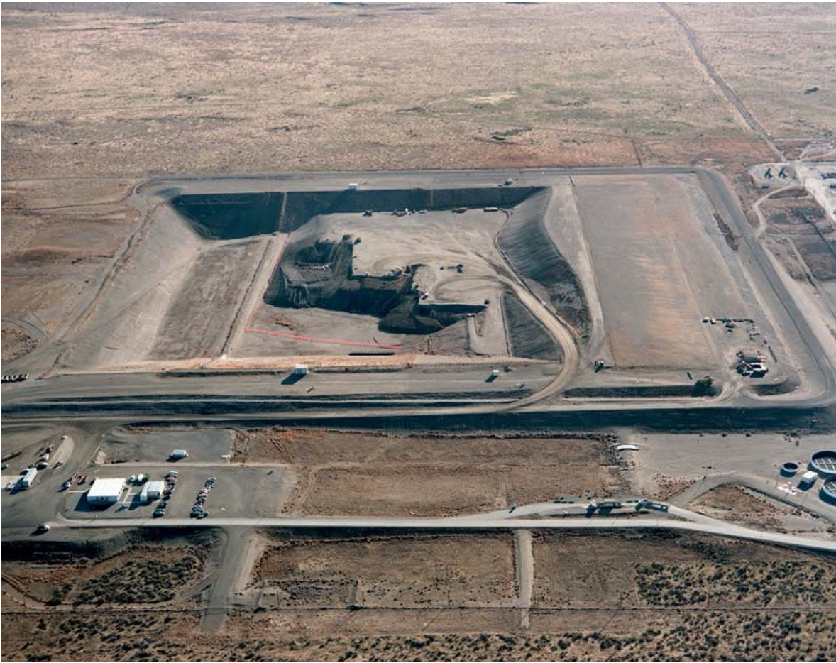
12 13 14 Figure 2.16. Environmental Restoration Disposal Facility (ERDF) 15
