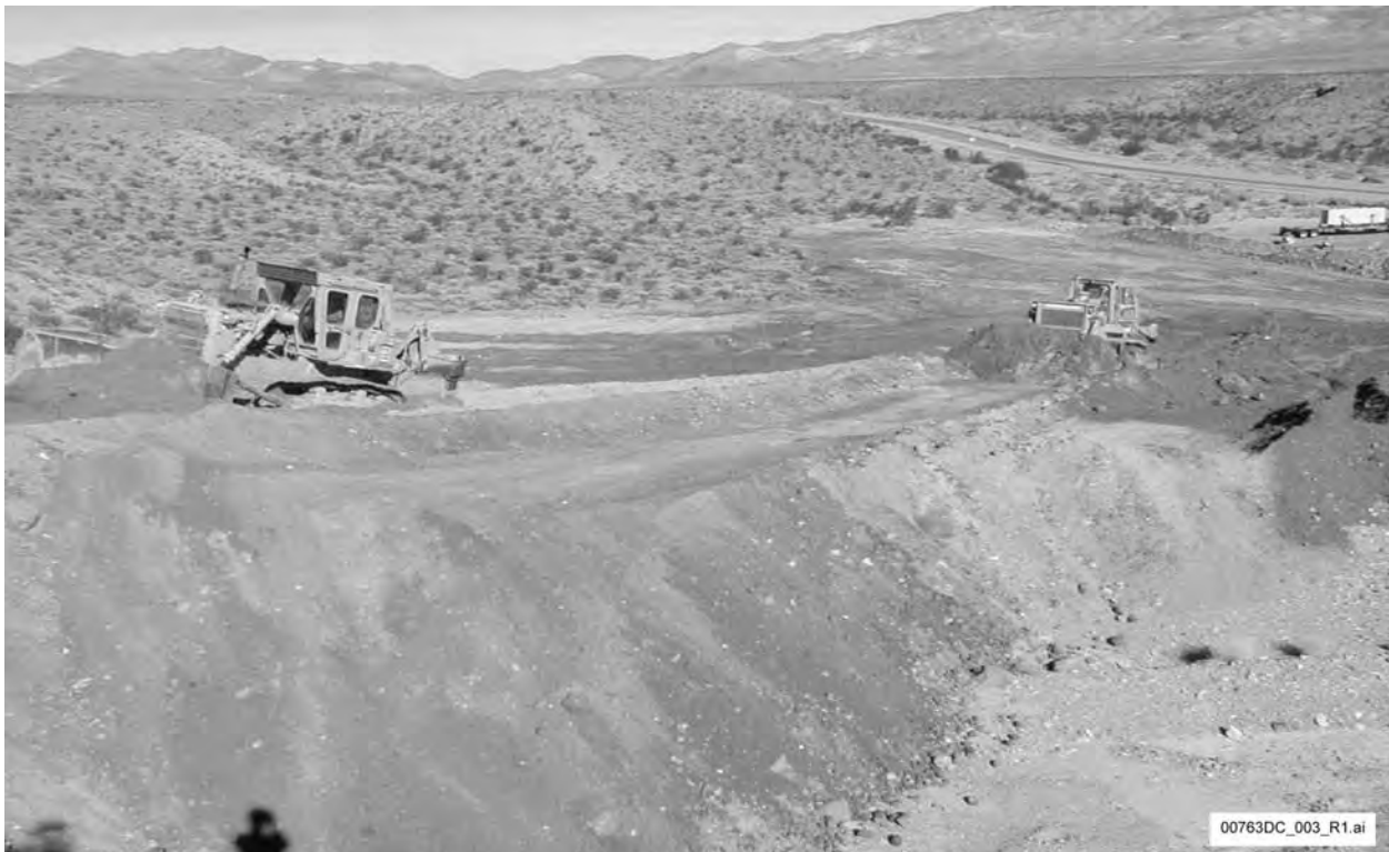
Figure 4-2. Fill material is spread and contoured on the site of a decommissioned borrow area at Yucca Mountain.
