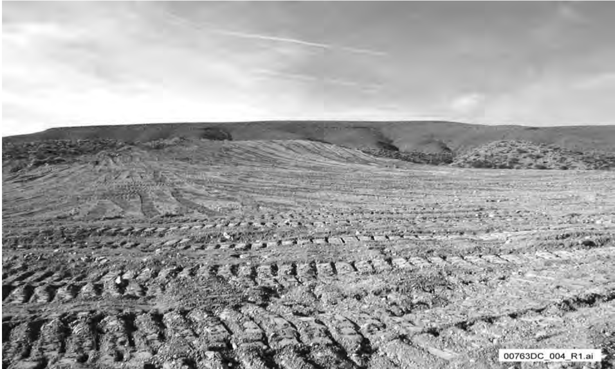
Figure 4-3. Decommissioned borrow area at Yucca Mountain that has been recontoured prior to seeding and mulching.
