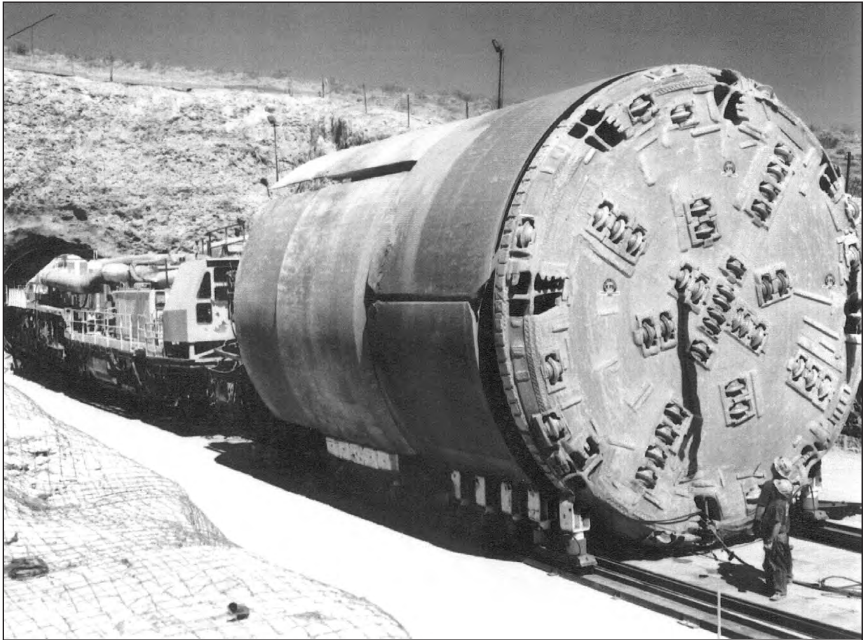
Figure 2-17. Tunnel boring machine.
