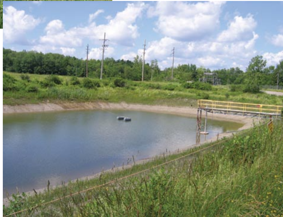
Lagoon 3. Storage Basin for Treated Wastewater Awaiting Discharge to Erdman Brook through the State Pollutant Discharge Elimination System (SPDES) - Permitted Discharge.
