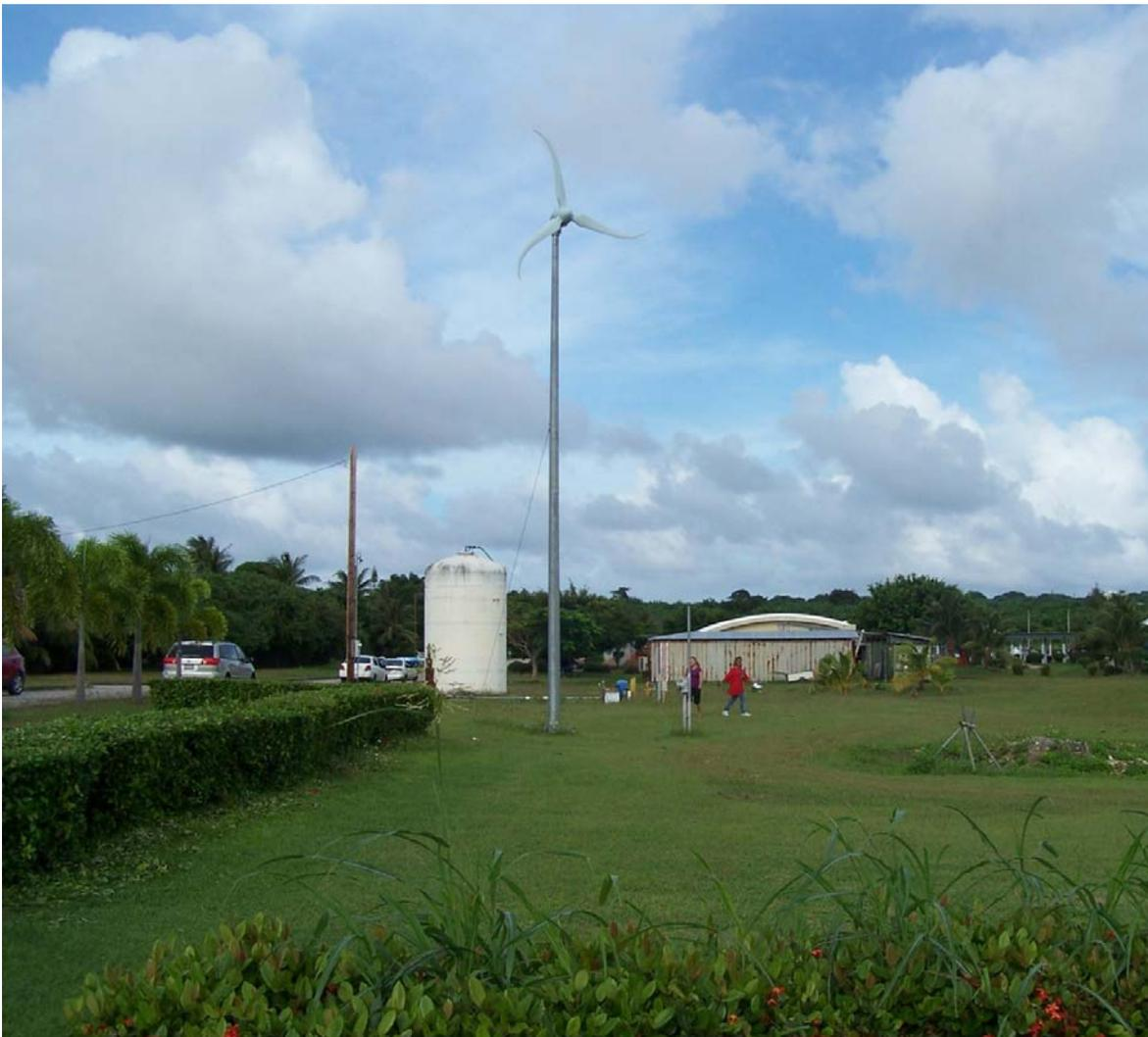
Figure 2. Skystream 2.4 kW wind turbine
