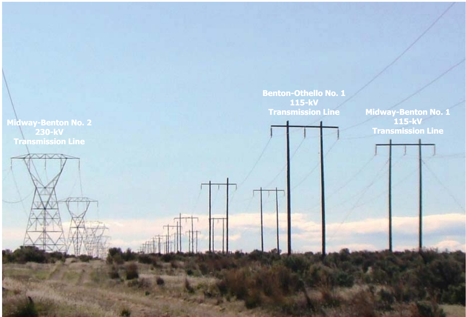
Figure 2-3. Existing Transmission Line Corridor
