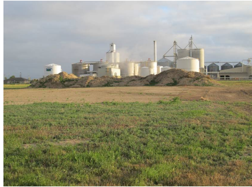
2) Looking north-northwest across the site showing dirt pile on the site, and the existing facility in the background.
