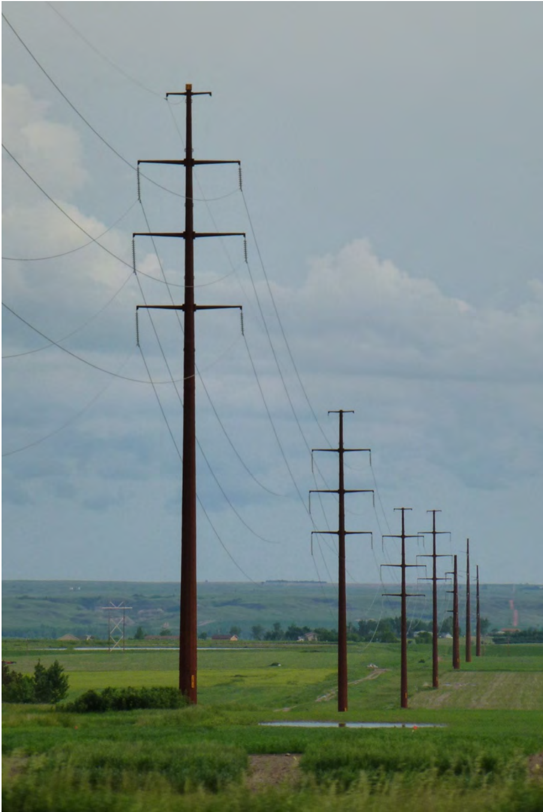
Figure 2.3-3 Single Pole Double circuit 230/115-kV Structure
