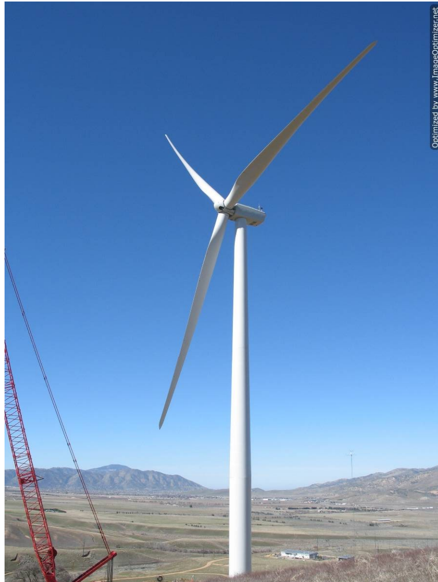
Figure 3-5. Photo of GE 1.6 100 Wind Turbines in an Industrial Wind Facility Setting
