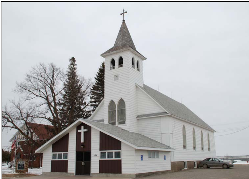
FIGURE 27. ST. ANN'S CATHOLIC CHURCH (MH-WBC-004), FACING NORTHEAST
