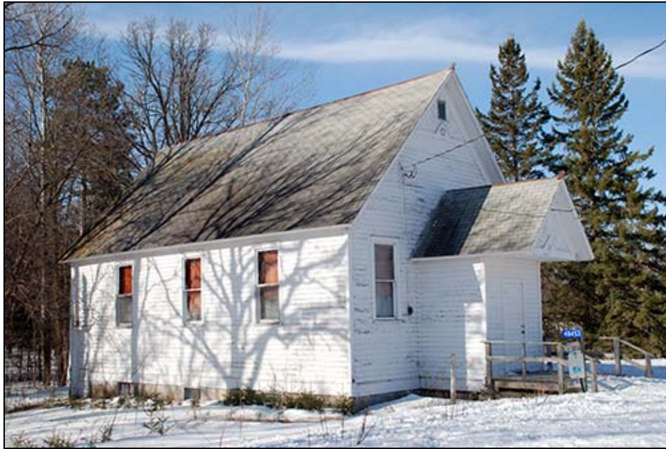
FIGURE 12. PONSFORD COMMUNITY CHURCH (BK-CAR-007), FACING SOUTHWEST
