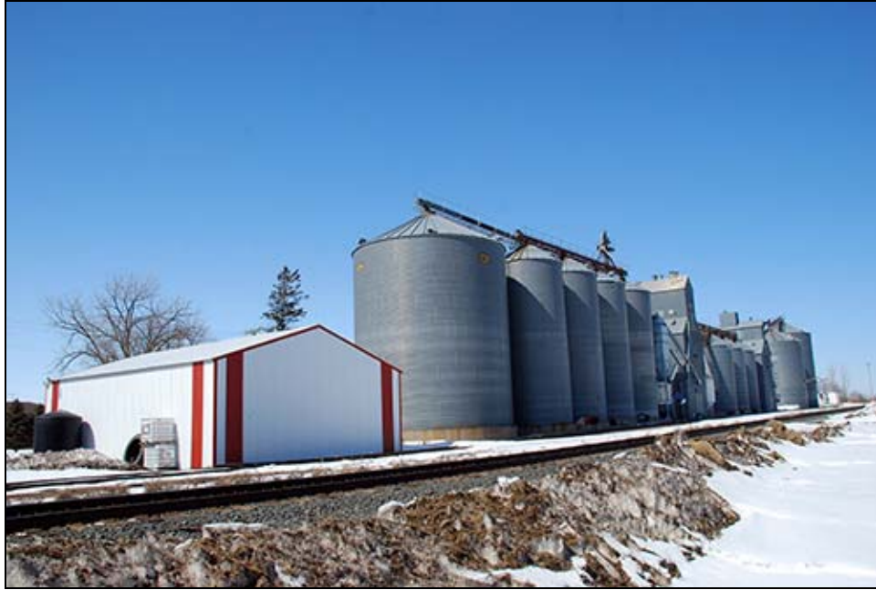
FIGURE 38. WAUBUN ELEVATOR COMPANY COMPLEX (MH-WBC-093), FACING NORTHWEST
