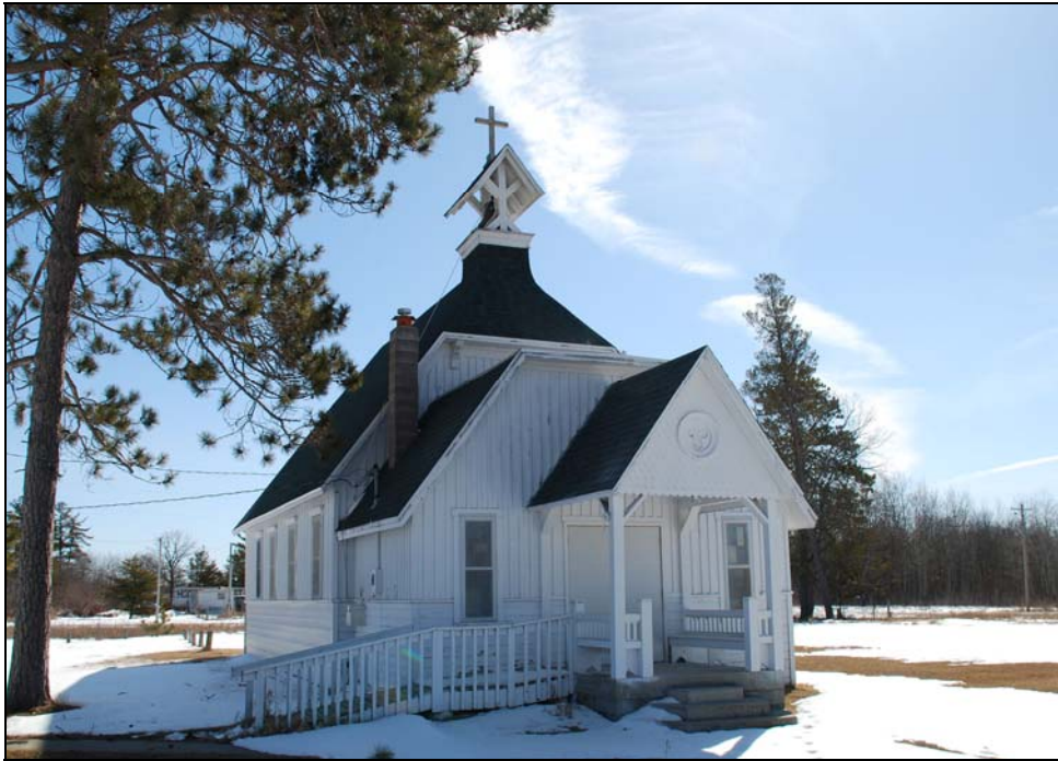
FIGURE 22. BRECK MEMORIAL EPISCOPAL CHURCH (BK-PNP-007), FACING SOUTHEAST
