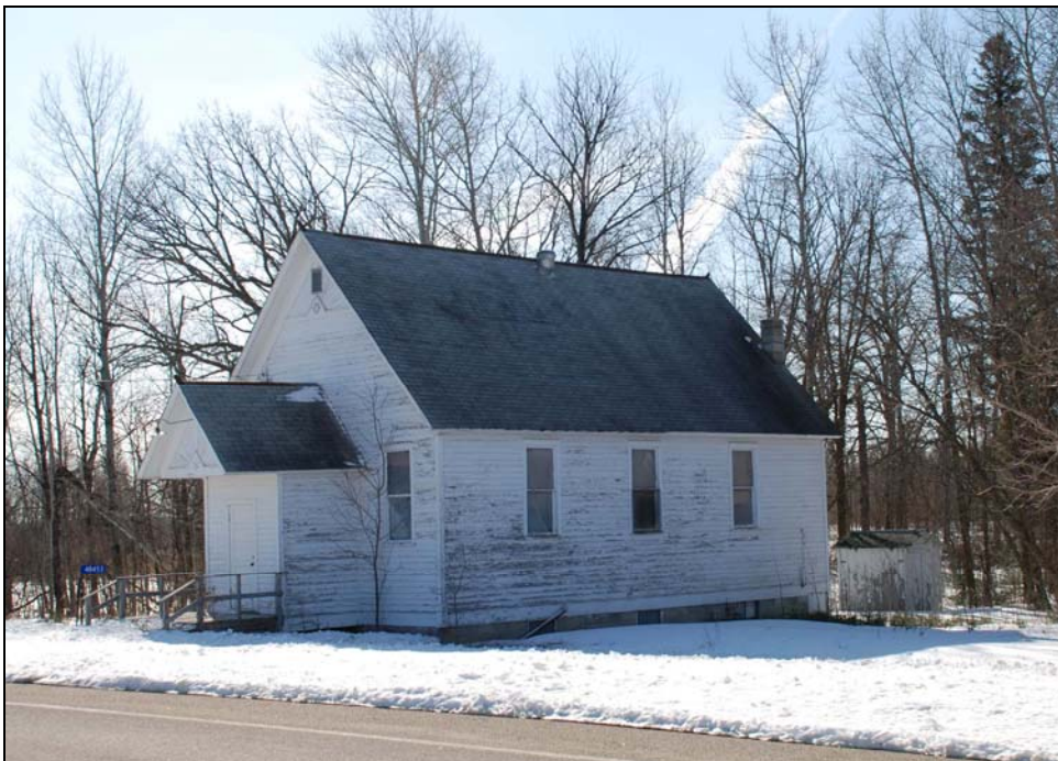
FIGURE 13. PONSFORD COMMUNITY CHURCH (BK-CAR-007), FACING SOUTHEAST
