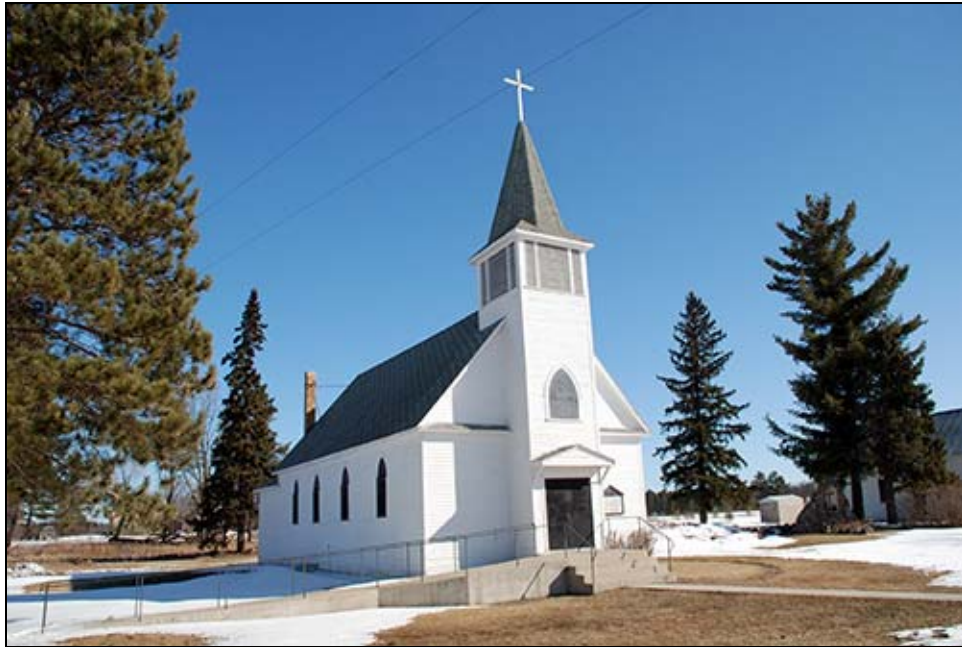
FIGURE 15. ST. THEODORE'S CATHOLIC CHURCH (BK-PNP-001), FACING NORTHEAST
