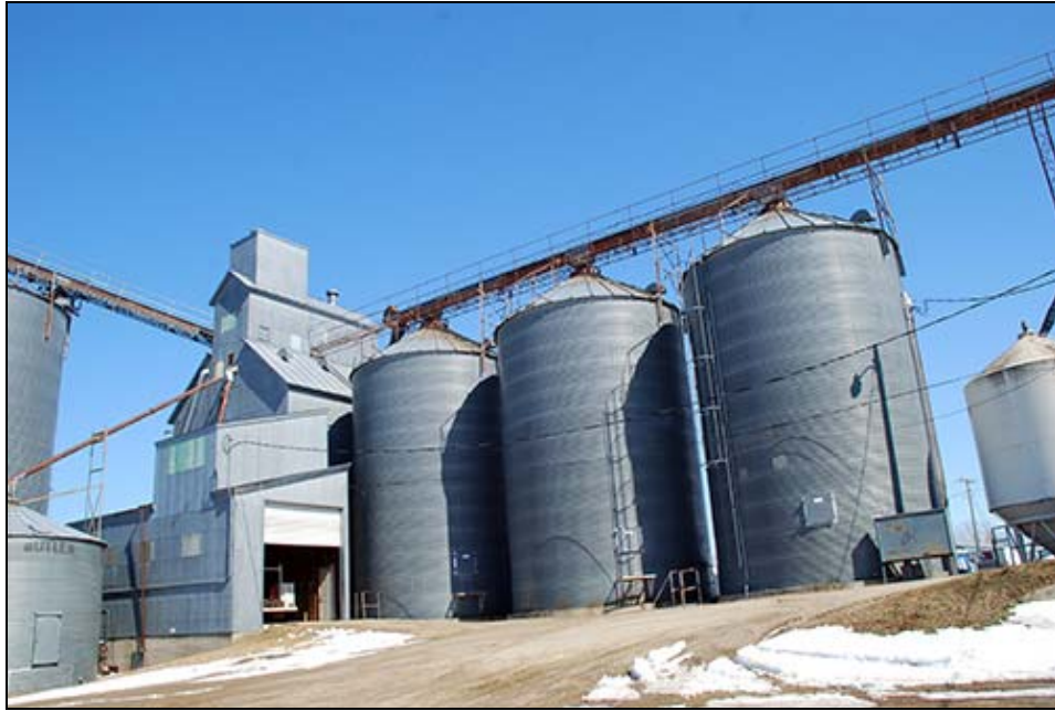
FIGURE 35. WAUBUN ELEVATOR COMPANY COMPLEX (MH-WBC-093), FACING NORTHEAST
