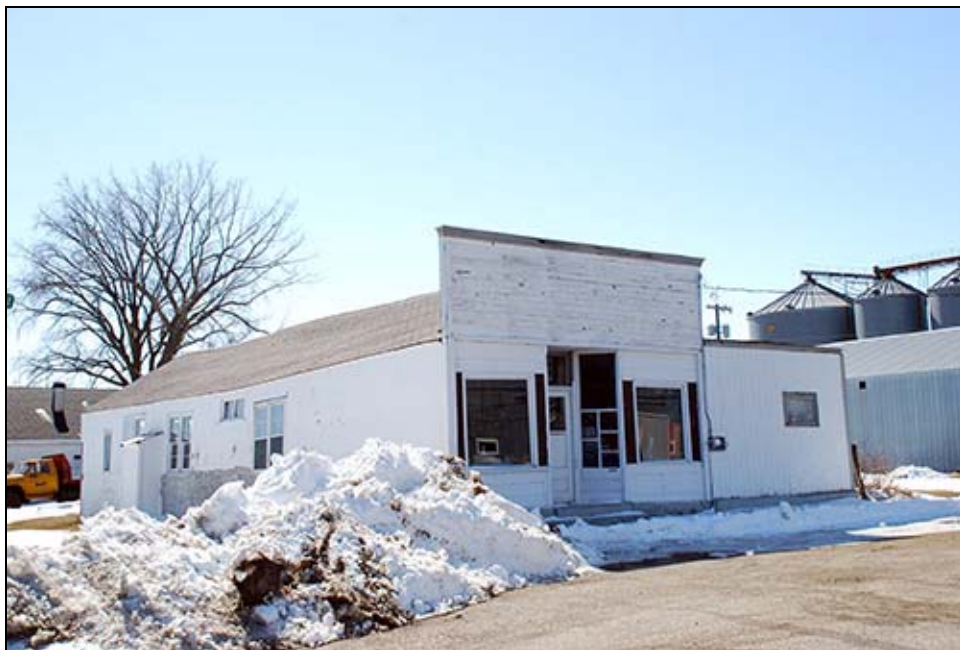
FIGURE 8. GOLDEN RULE STORE (MH-WBC-078), FACING SOUTHWEST
