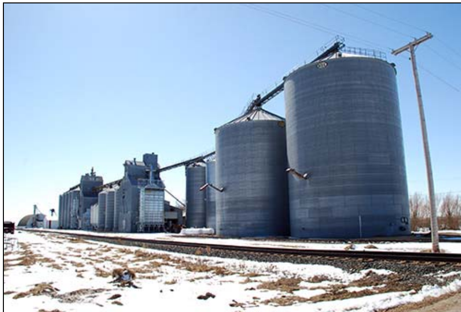
FIGURE 34. WAUBUN ELEVATOR COMPANY COMPLEX (MH-WBC-093), FACING SOUTHWEST
