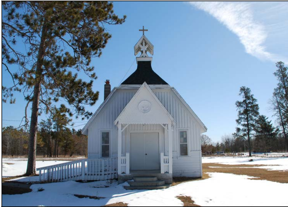
FIGURE 23. BRECK MEMORIAL EPISCOPAL CHURCH (BK-PNP-007), FACING EAST
