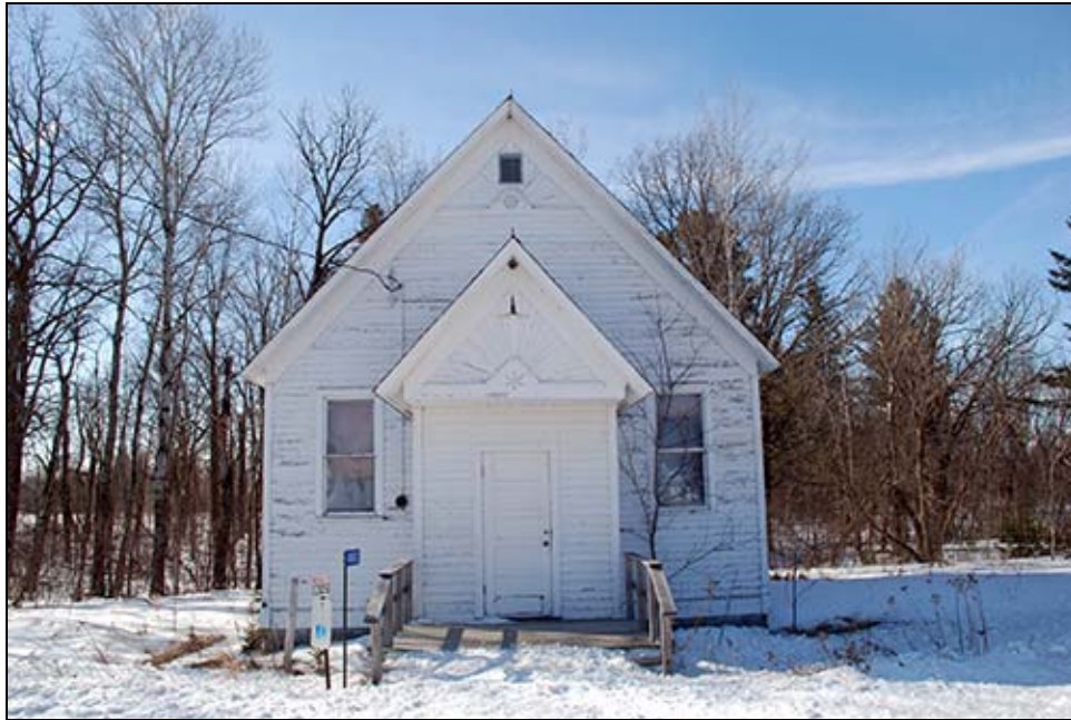
FIGURE 14. PONSFORD COMMUNITY CHURCH (BK-CAR-007), FACING SOUTH
