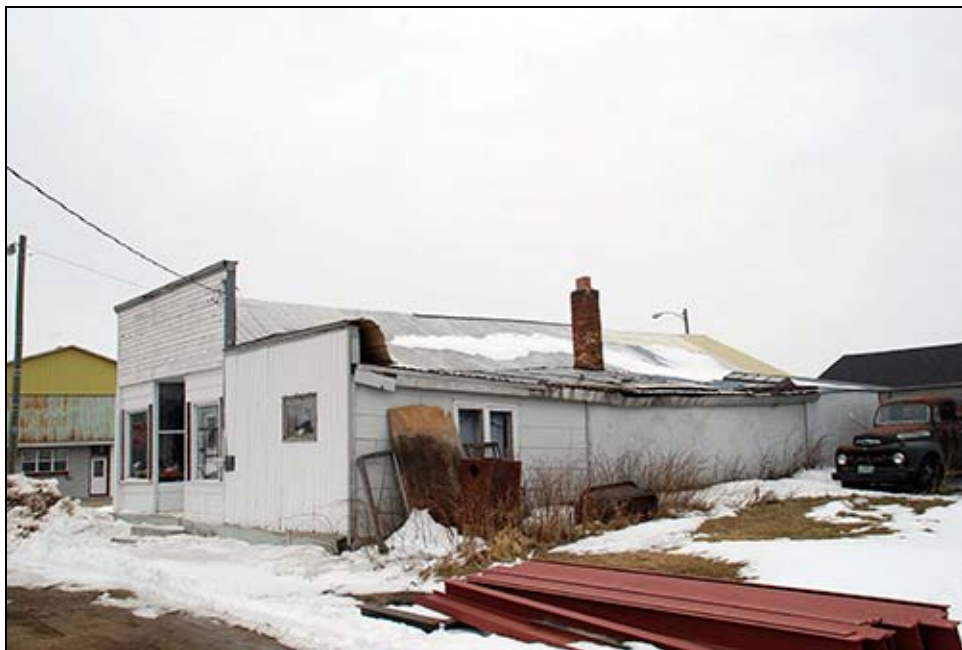
FIGURE 10. GOLDEN RULE STORE (MH-WBC-078), FACING SOUTHEAST
