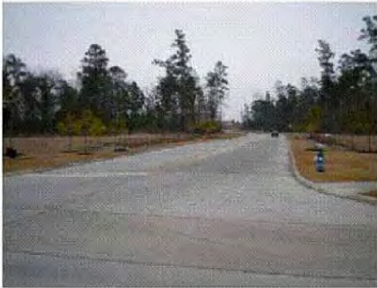
Figure 8. Looking northward at Waterbend Cove Road.
