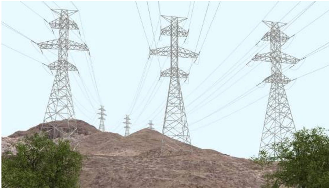
Figure 3-22. Computer-simulated view from the Visitor’s Center upper parking lot oriented westward with the proposed transmission lines proposed by the Preferred Alternative.
