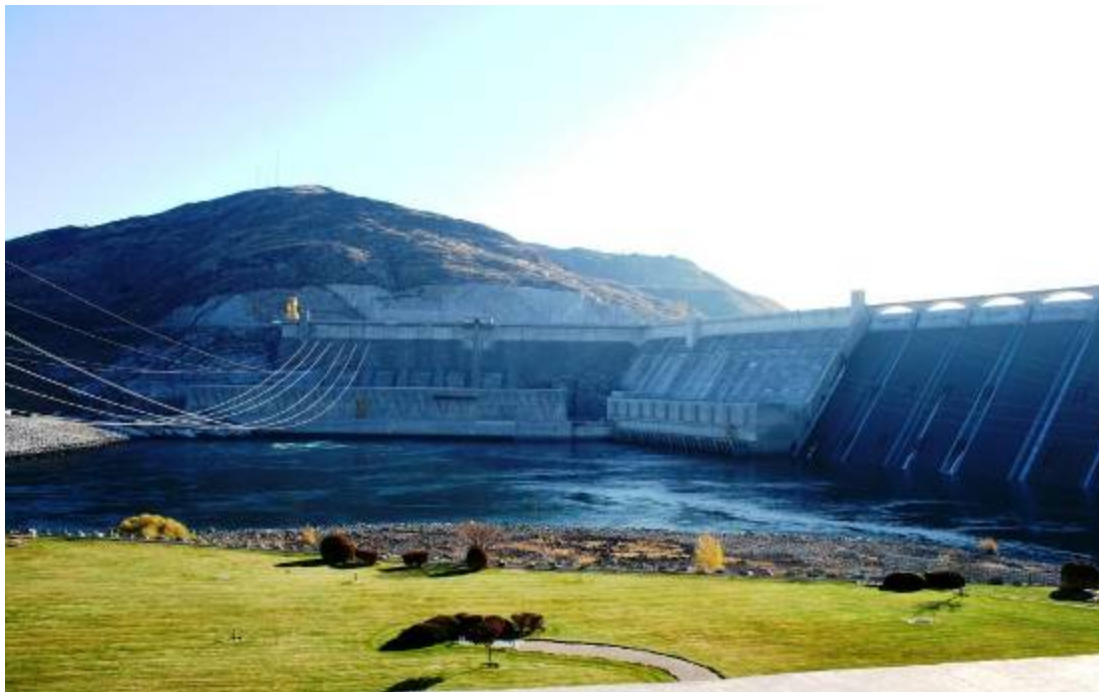
Figure 3-18. View of Grand Coulee Dam from the Visitor Center parking lot. (Note the backup transmission lines on the left-hand side of the photo)
