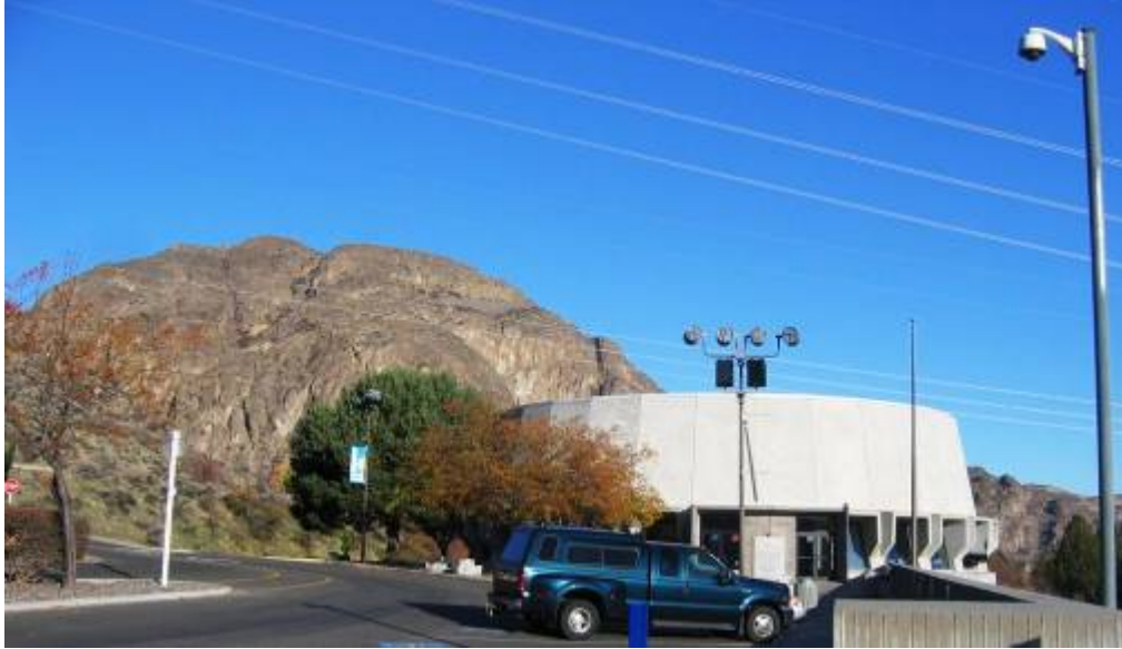
Figure 3-20. The entrance to the Visitor's Center upper parking lot. ( Note the backup transmission lines that currently span over the Visitor's Center )
