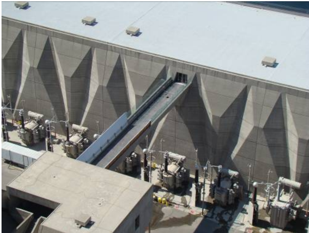
Figure 3-8. Tour bridge that connects the Incline Elevator to the TPP, which will be removed as part of the Proposed Action.
