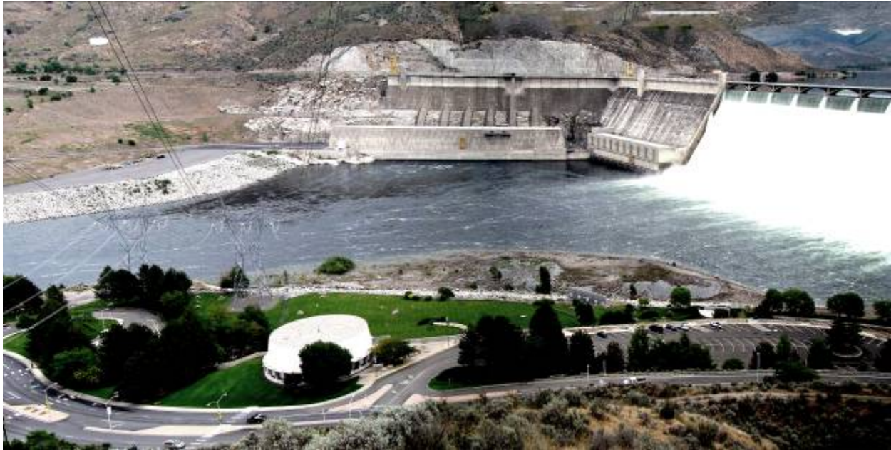
Figure 3-10. The Grand Coulee Dam with views of the TPP, the Visitor's Center, and the backup overhead lines that span above the Visitor's Center.
