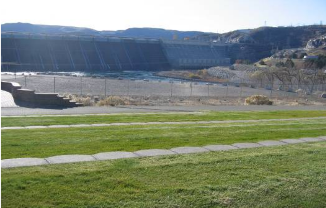
Figure 3-27. View of Grand Coulee Dam from Freedom Point..
