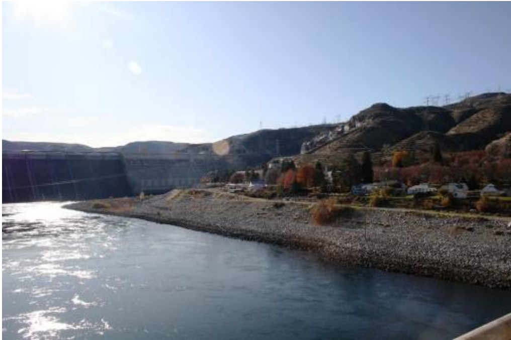
Figure 3-16. Approaching the City of Coulee Dam from the North as seen from the Grand Coulee Columbia River Bridge.
