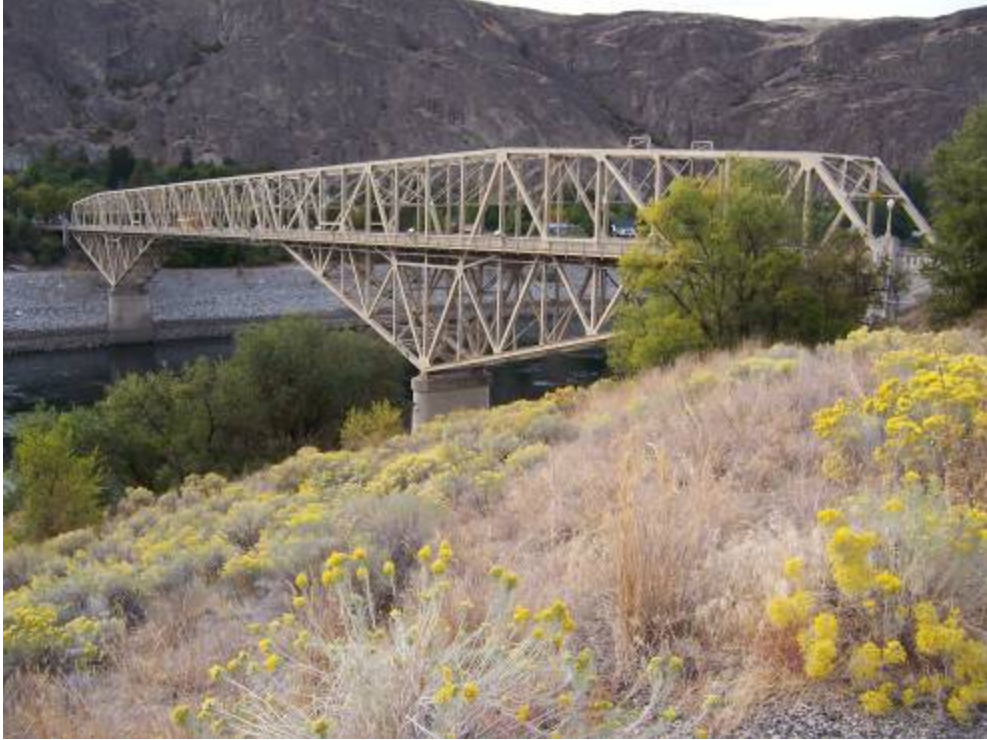
Figure 3-15. The Grand Coulee Columbia River Bridge.
