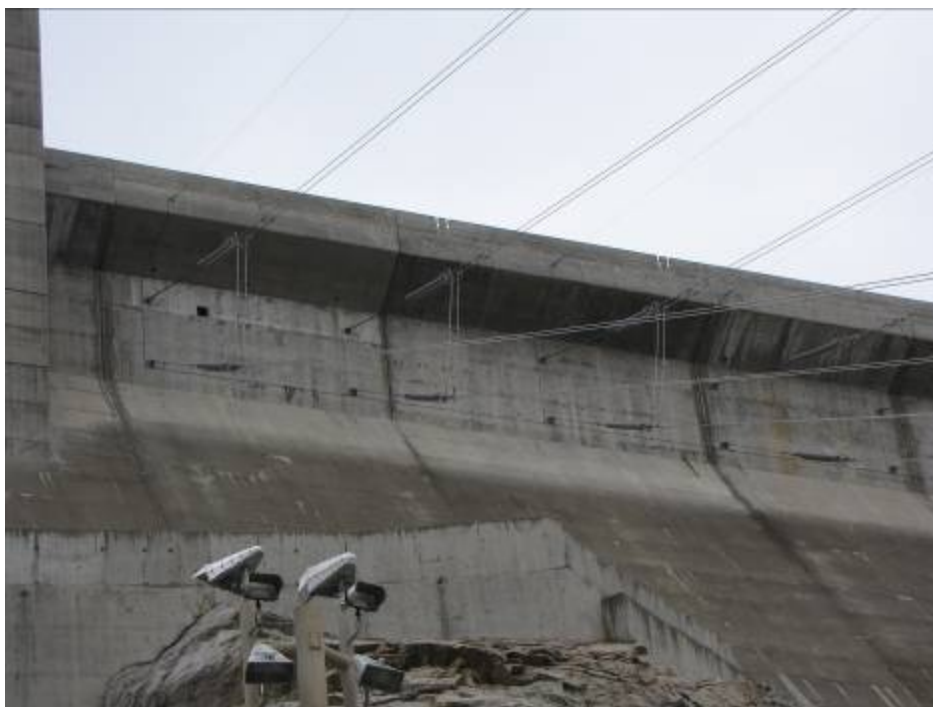
Figure 3-34. Current anchoring of the backup lines to the Forebay dam.
