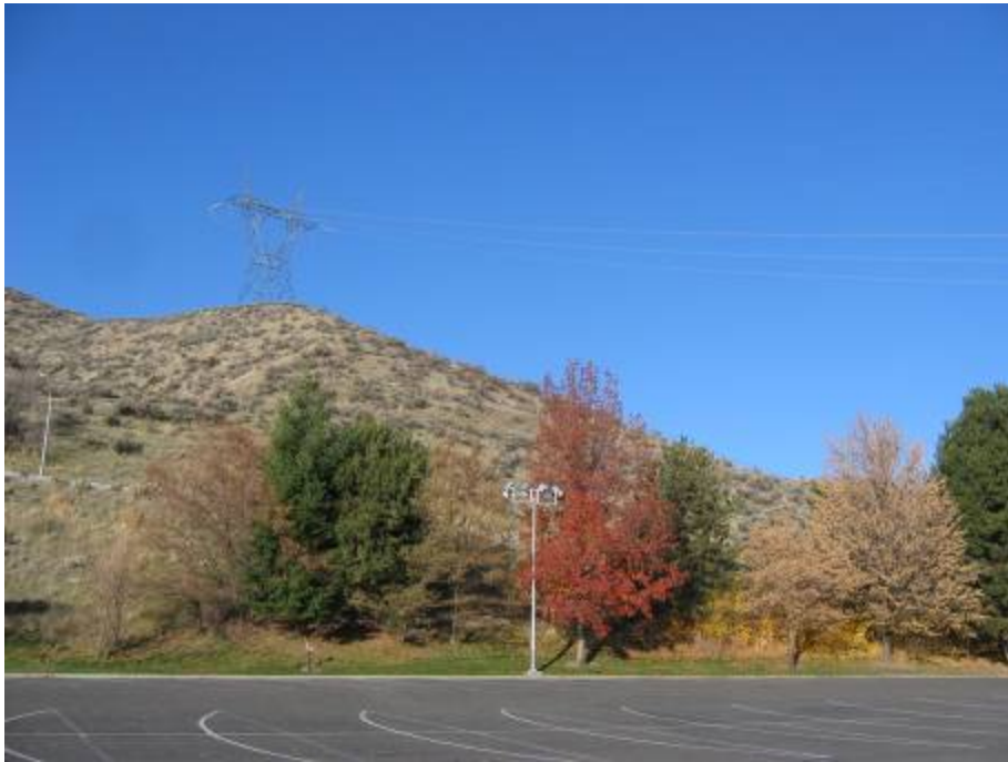
Figure 3-21. View of the existing backup towers looking west from the Visitor's Center.
