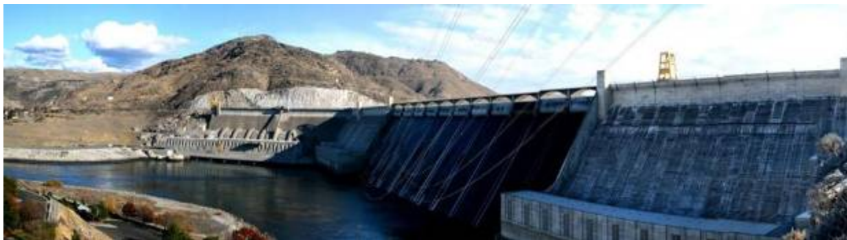
Figure 3-13. View of the Grand Coulee Dam from the SR 155 Turnout Viewpoint.
