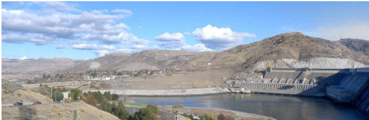
Figure 3-14. Northbound Viewpoint into the City of Coulee Dam on SR 155.
