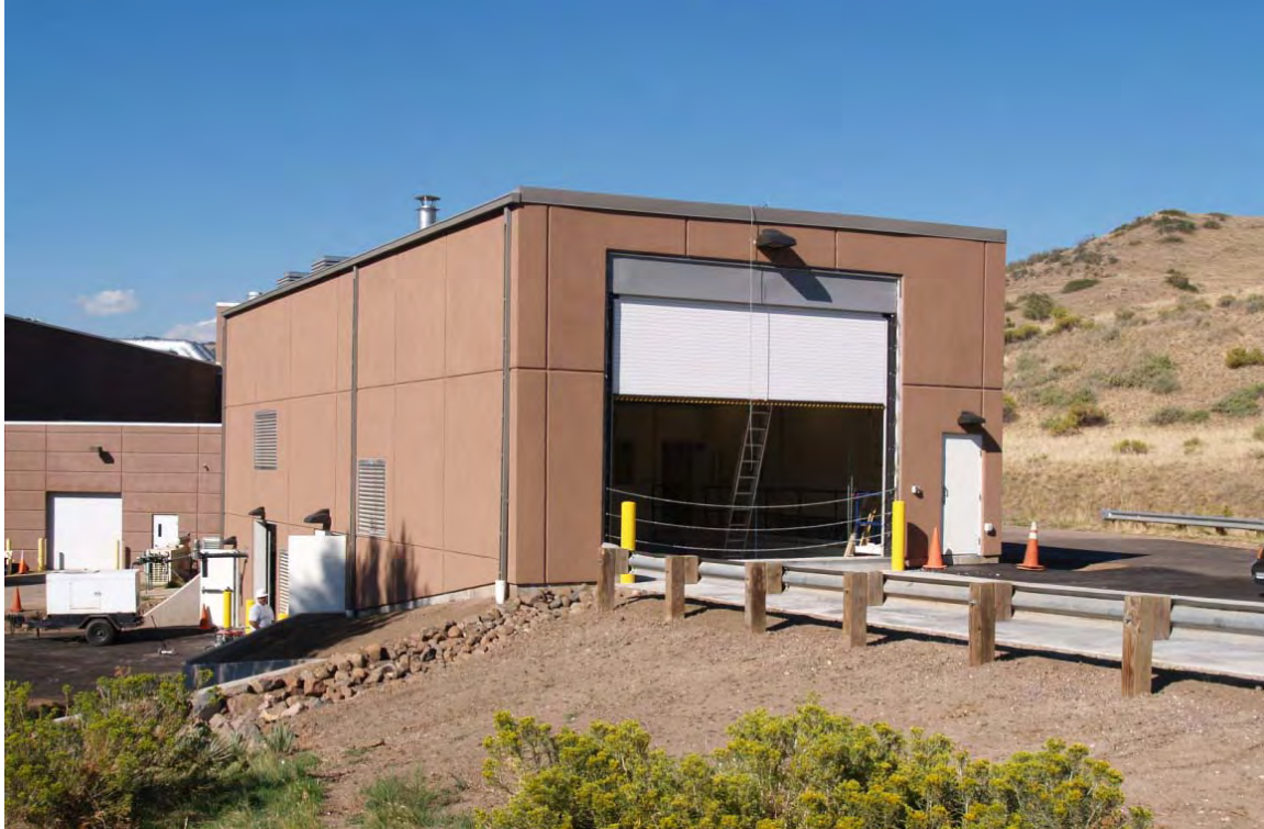
Figure 2-3. View of the east side of the RFHP at the unloading area for woodchips. Open bay door leads to the fuel pit. Proposed silo would be located on the asphalt area to the left and below the building.
