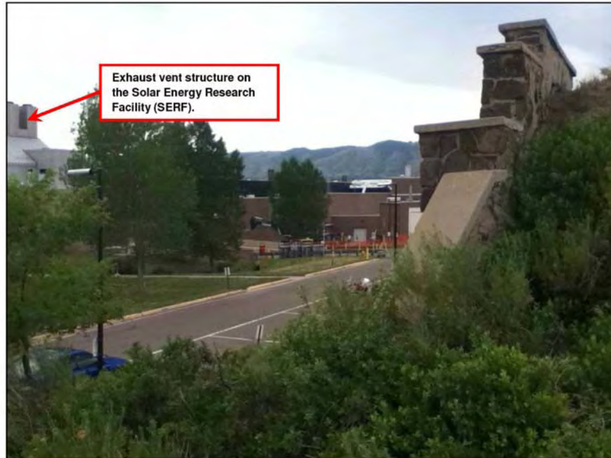
Photo 5. View from Ammunition Igloo to the southwest toward the RFHP. From this perspective, the proposed RFHP silo would appear smaller than the existing exhaust vent structure on the Solar Energy Research Facility.
