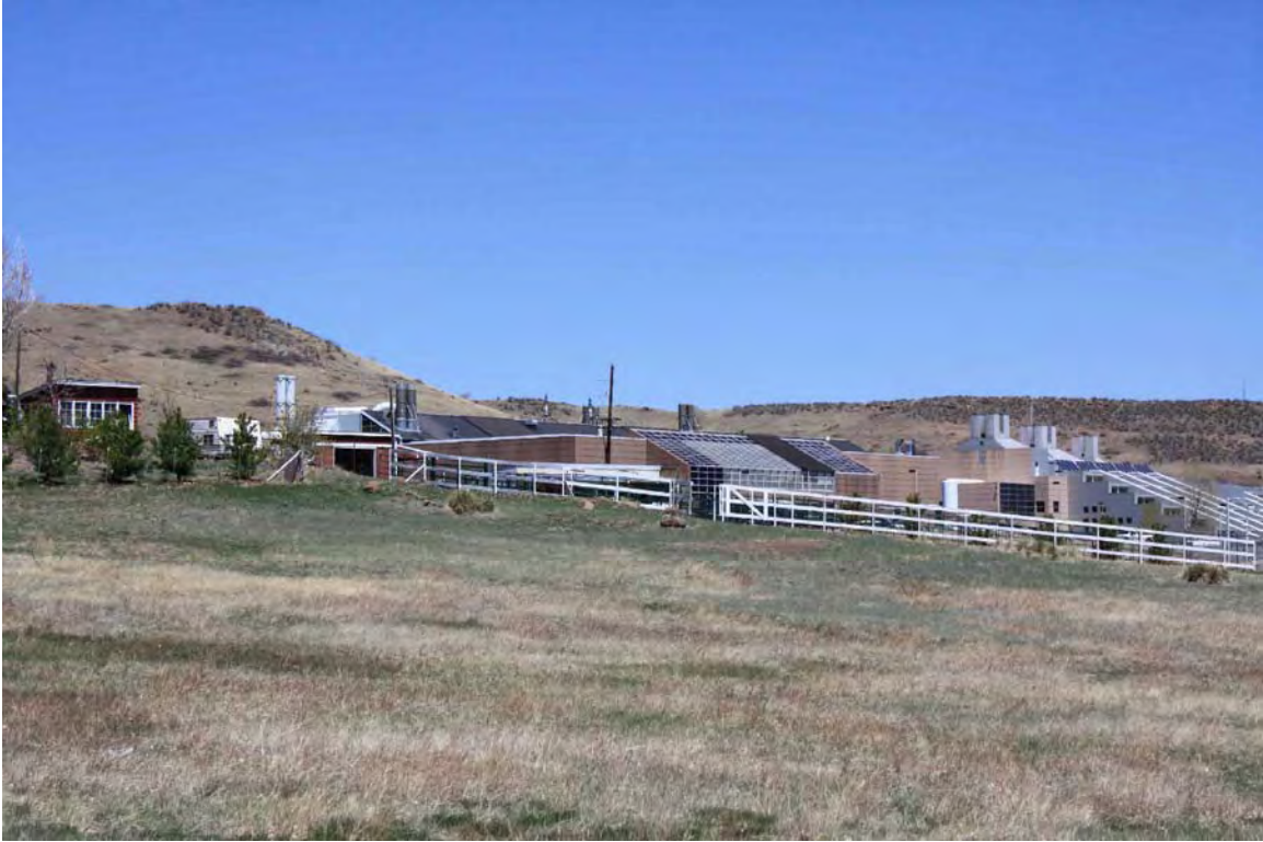
Figure 3-2. Current view of the STM site in April 2011 as seen from the intersection of Nile and Moss streets.
