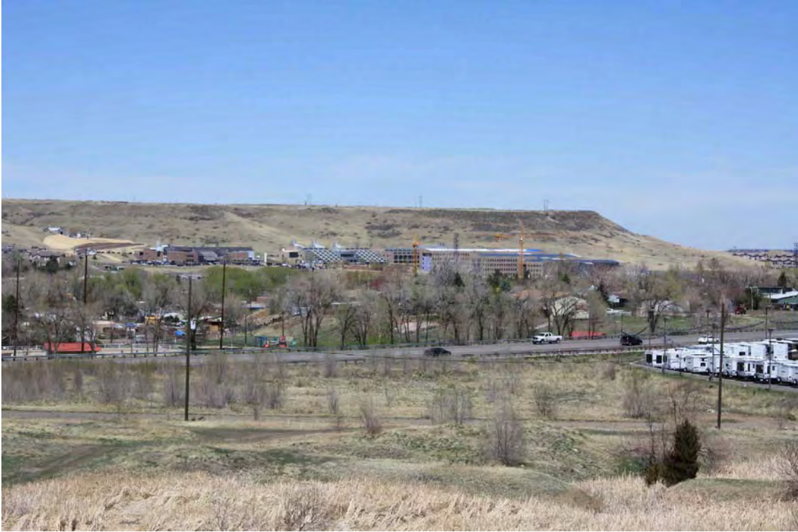
Figure 3-4. Current view of the STM site in April 2011 as seen from the U.S. Highway 6 exit ramp westbound to I-70.
