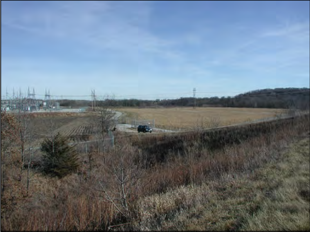
Figure 10. OGS Substation and Typical Surrounding Landscape
