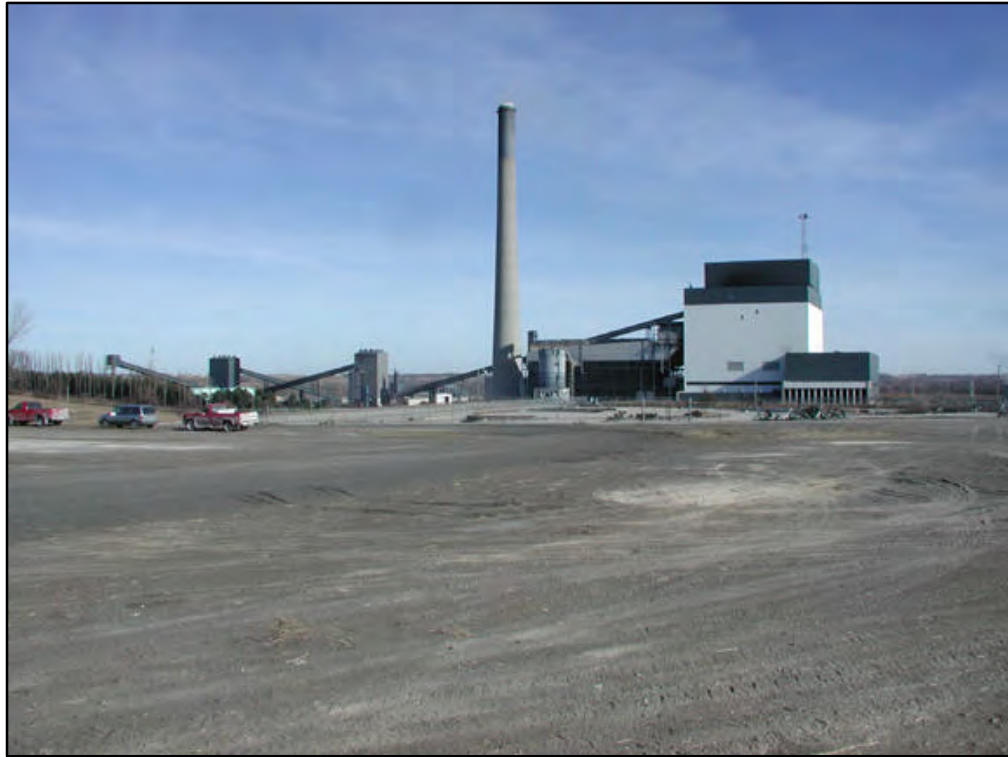
Figure 3. OGS Plant Looking Northeast from the Site of the Proposed New Facilities
