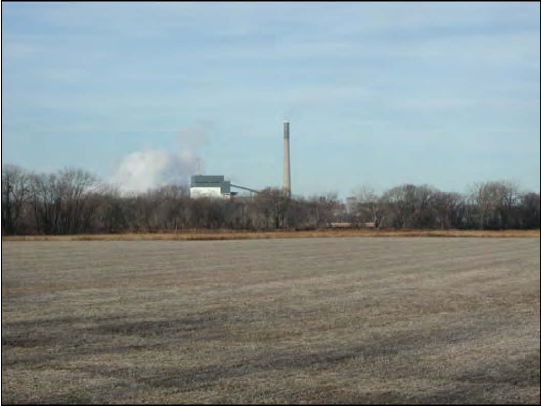
Figure 11. OGS Plant from the East
