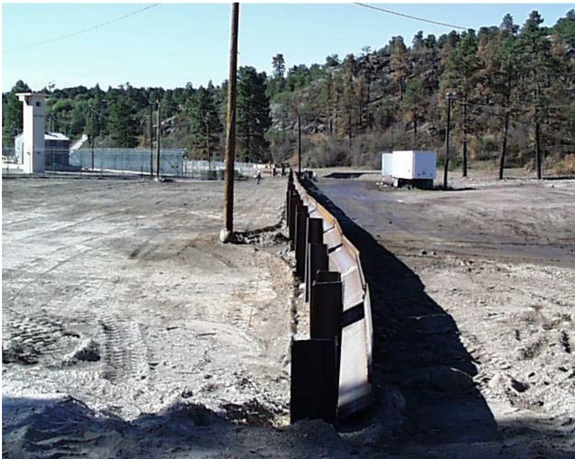
Figure 13. Steel diversion wall at TA-18 under construction.
