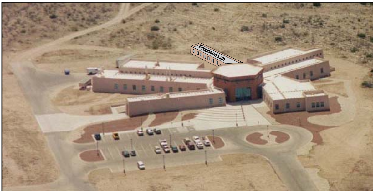
Figure 1-2. Aerial View of the CEMRC and Proposed ACRSL Facility
