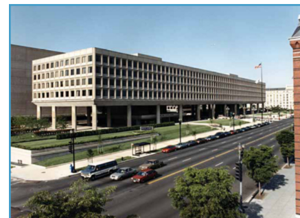
DOE Headquarters Forrester Building in Washington, D.C.
