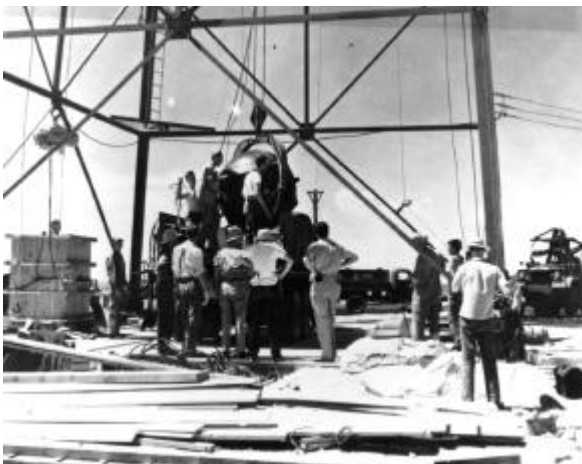
Trinity device being readied. Source: Department of Energy.
