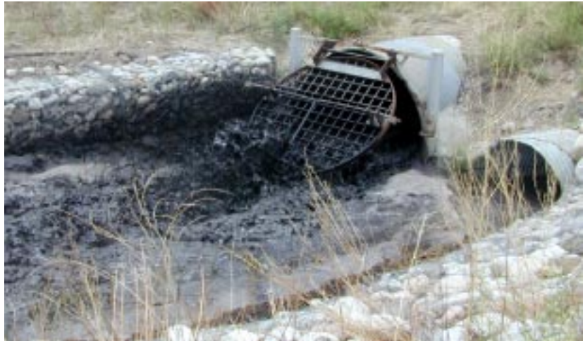
Post-fire runoff, shown here emerging from a culvert, is now black with soot.
