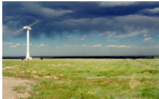
The site-wide EA evaluated the impacts of adding more test turbines like this one at the site.
