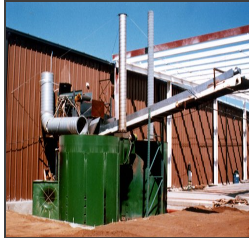
Biomass Heat Exchanger NREL/PIX 03447
