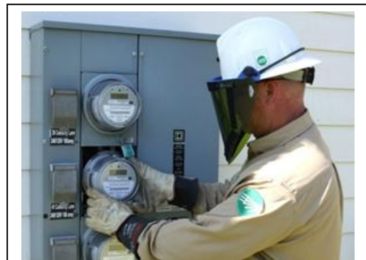
TEC technician changes-out an analog meter with a smart meter at a customer home.
