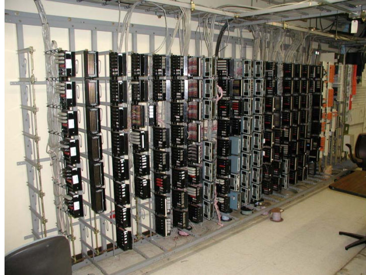
Plain old telephone service inside control center
