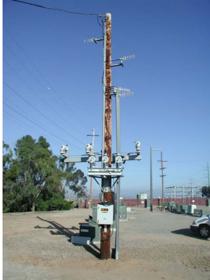
Field components with radio antennas
