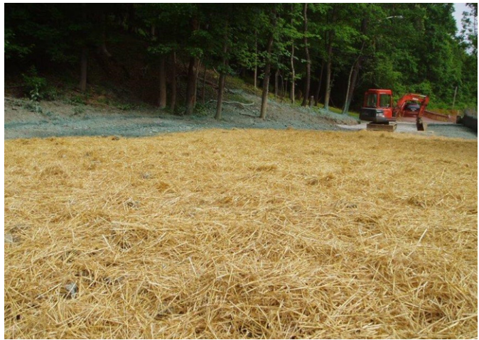
FIGURE 9 | NETL-Pittsburgh Site Water Line Project, vegetation restoration phase, June 2015
