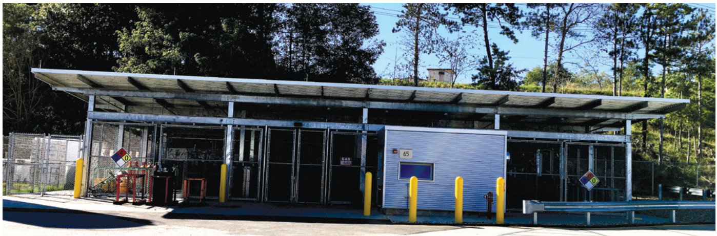
FIGURE 15 | Compressed gas cylinders at NETL-Pittsburgh
