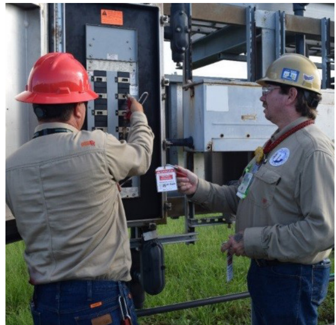
FIGURE 22 | The SPR West Hackberry site – Lockout-Tagout training, August 2017
