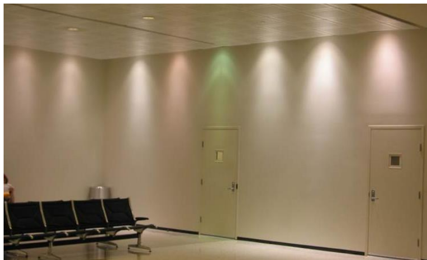
Figure 2. A room lit with ceramic metal halide lamps shows the impact of poor chromaticity stability on the appearance of the wall wash. The varying color appearance of neighboring lamps would necessitate relamping.
