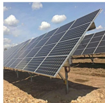
FIXED-TILT RACKING SYSTEM (TYPICAL) OR APPROVED EQUIPMENT
