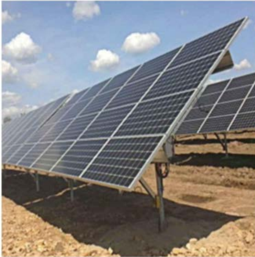
FIXED-TILT RACKING SYSTEM (TYPICAL)
