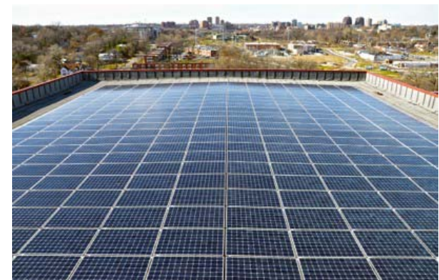
180 kWh solar at 8 locations (including local High School)
