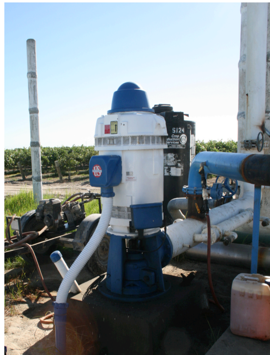
An irrigation pump connected to a web-to-wireless controller designed by M2M Communications.
