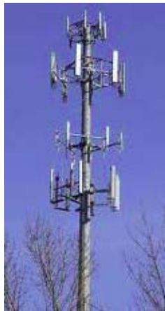
Figure 2.4.3-1: Monopole Cell Tower with Multiple Panel Antennas
