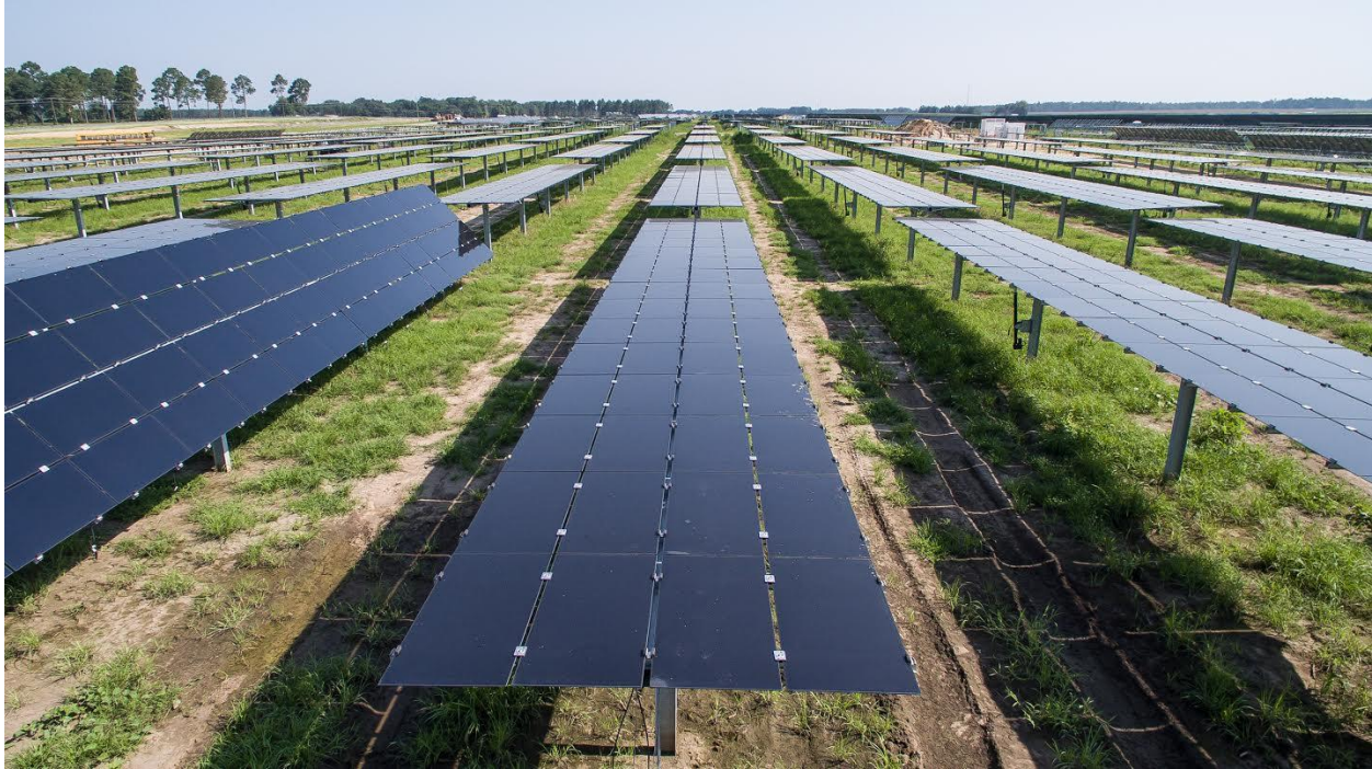
Figure 3.4 Example of smooth glass solar panels without an arc.
