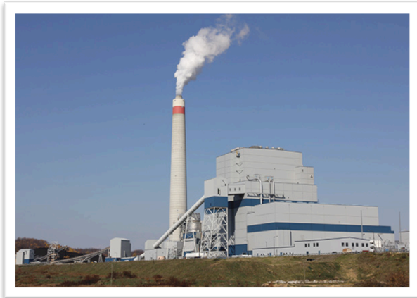
Figure 2: Longview Power Plant
