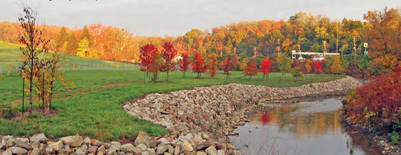
Canonsburg, Pennsylvania, Disposal Site.
