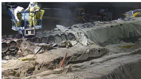
Photo on top was taken in 1978 and shows original stacking of drums filled with TRU waste. Notice the plastic wrapping. Photo below was taken on Aug. 23, 2016, showing technicians removing the original plastic wrap.
