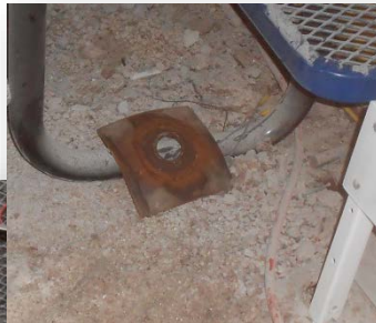
Roof bolt plate
