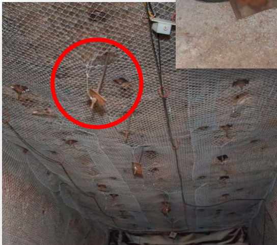
Broken roof bolts
