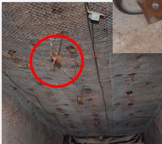
Broken roof bolts
