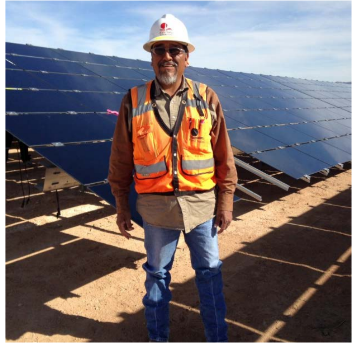
Photo of Anthony Frank, member of the Moapa Band of Paiutes and supervisor on the First Solar trenching team at the Moapa Southern Paiute Solar Project.
