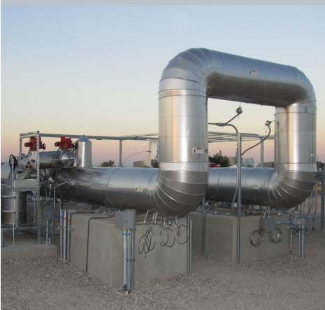
This molten salt test loop at Sandia National Laboratories' National Solar Thermal Test Facility has been used to further understand challenges related to thermal energy storage. Photo Courtesy: Sandia National Laboratories
