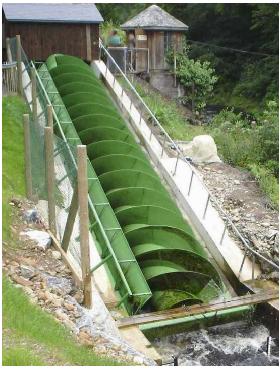
Figure 1-8. Archimedes screw for hydropower generation
