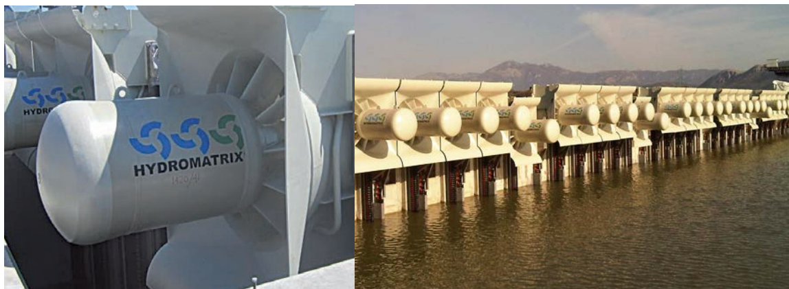
Figure 1-10. Modular application of standard turbine runners to an existing dam
