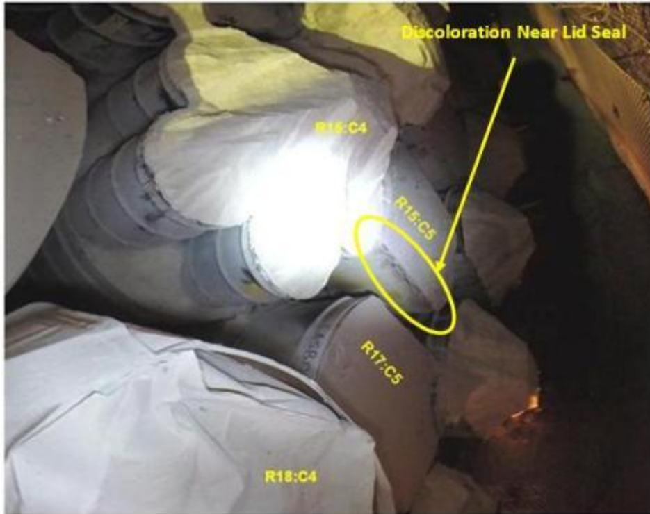
Figure 6-35: Discoloration of SWB at R15:C5
