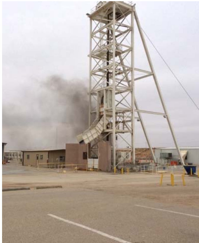
Figure 6-43: Upcasting Observed at the Salt Shaft on February 5, 2014
