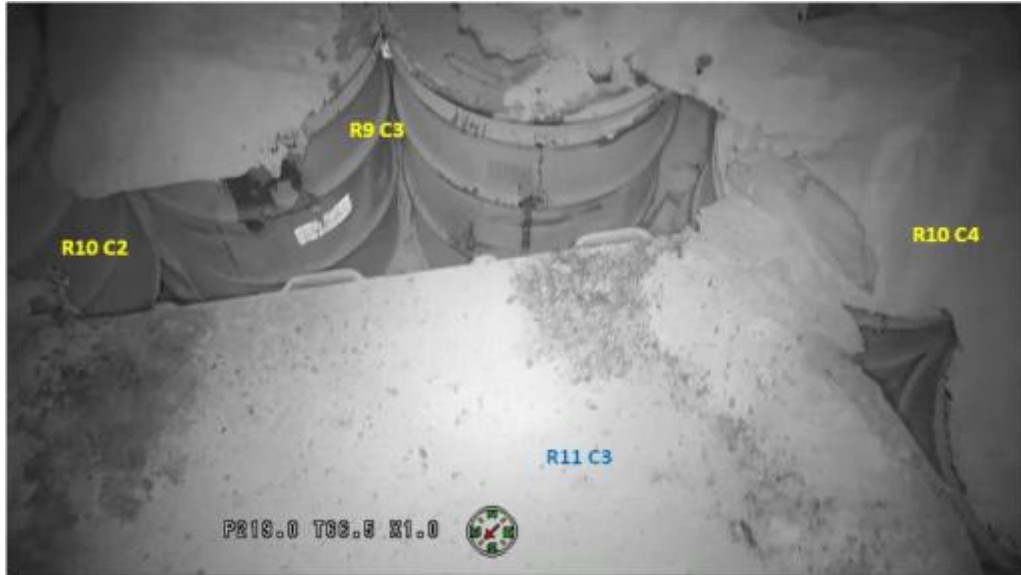
Figure 6-21: R9:C3 West Side
