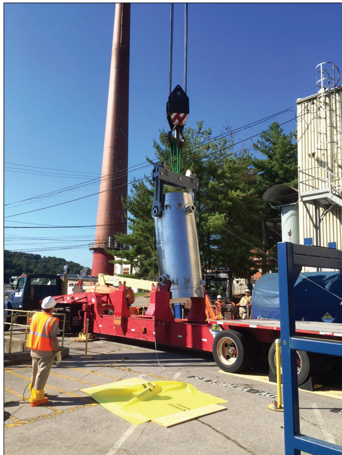
Workers load a cask containing irradiated components at the Oak Ridge Research Reactor, Building 3042.
