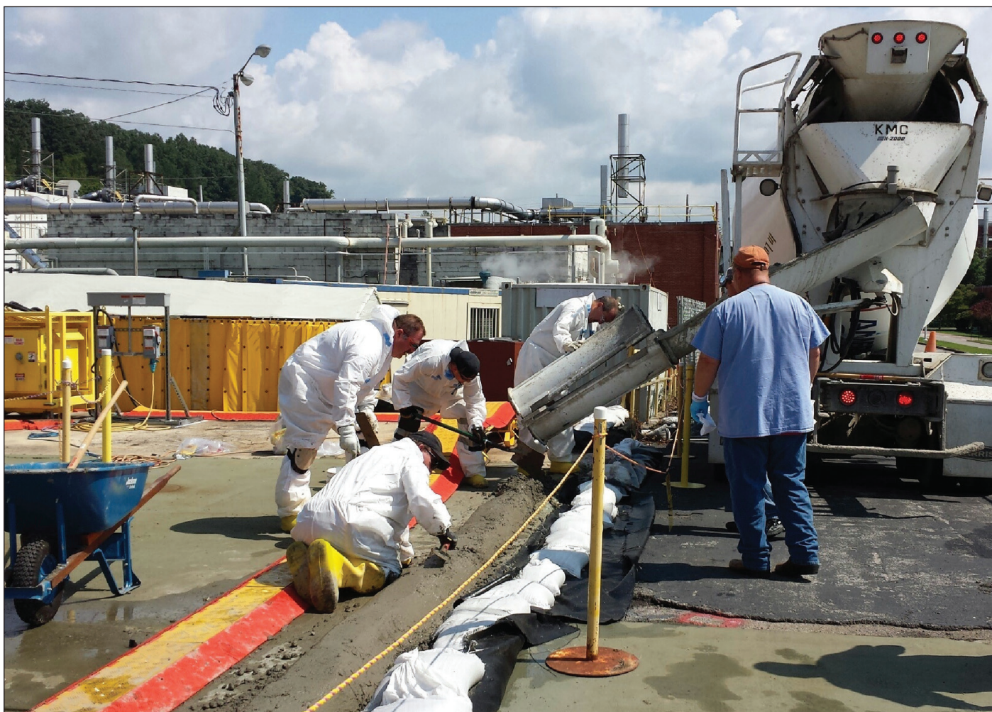
A concrete berm is being poured as part of the 3026 stabilization activities
