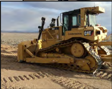
Central Nevada Test Area Site.
