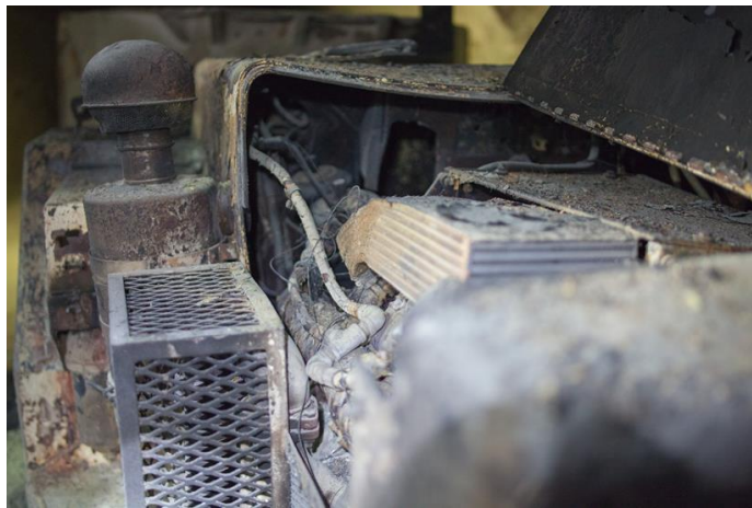
Figure 19: Engine Cooling Coils
