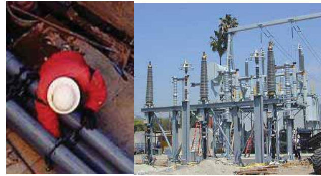
Underground Transmission Lines (P36)
