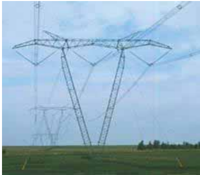
Overhead Transmission Lines (P35)
